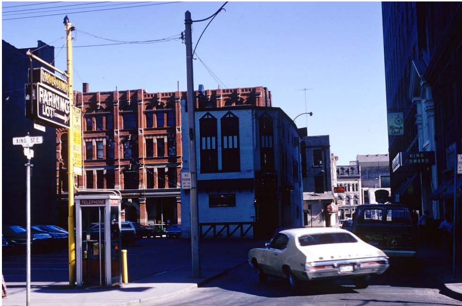
15. Archival Photographs, 40 Colborne Street, 1972 and 1973: showing the subject property at the northeast corner of Colborne Street and Leader Lane with the south entrance and St. James' Cathedral in the background (above), and from King Street East with the heritage properties at 45-55 Colborne Street in the background (below) (City of Toronto Archives, Series 841, Item 28 and Fonds 1526, Item 97).
