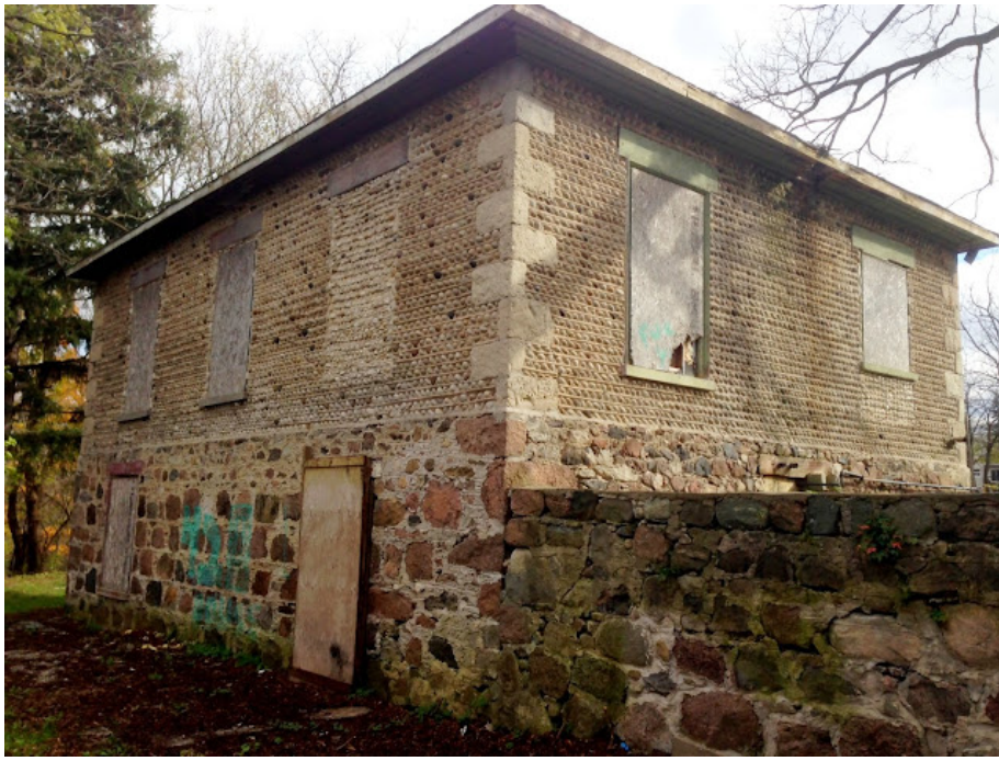
Rear, prior to restoration
