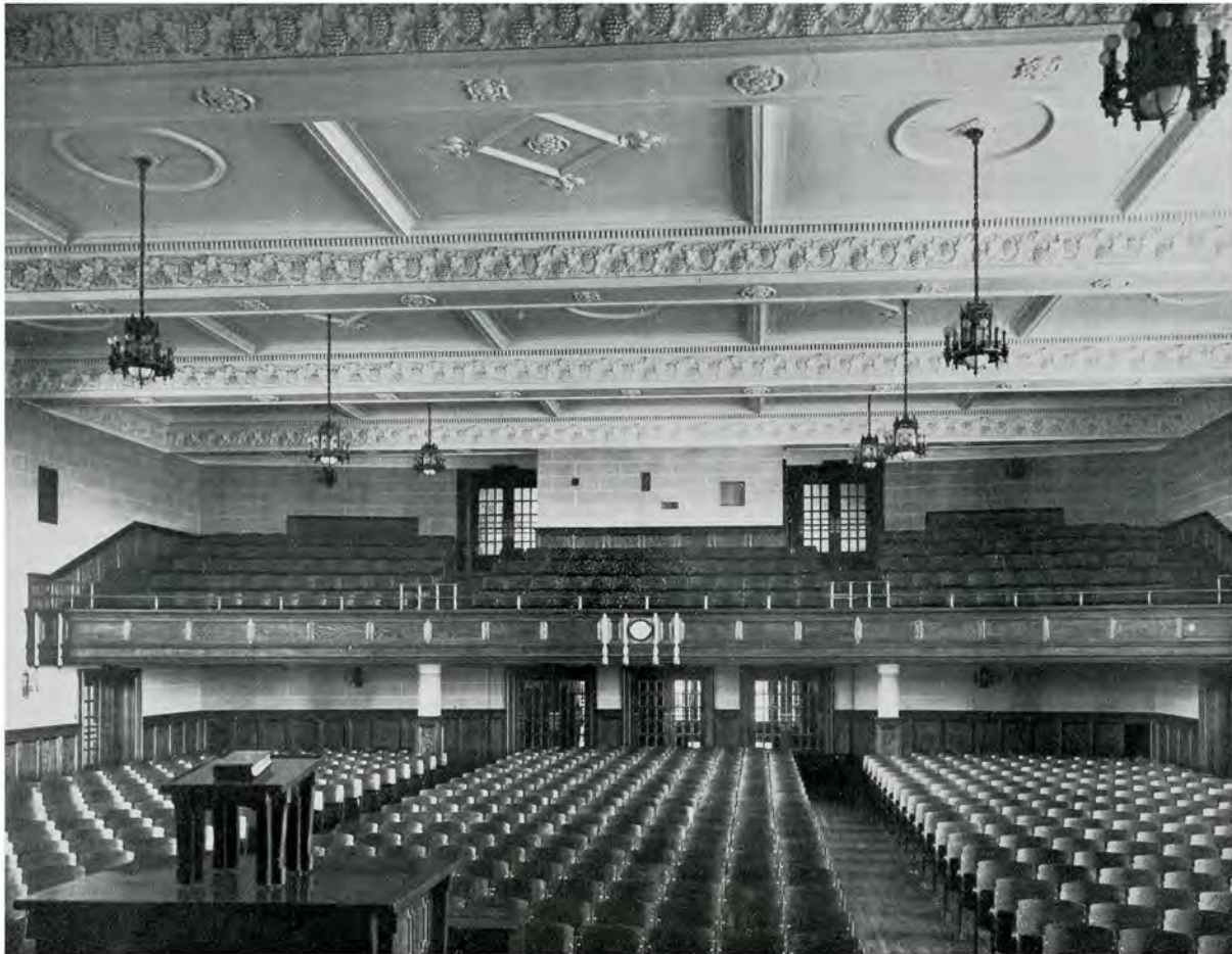
ASSEMBLY ROOM—RIVERDALE TECHNICAL SCHOOL Architectural Dept., Toronto Board of Education
