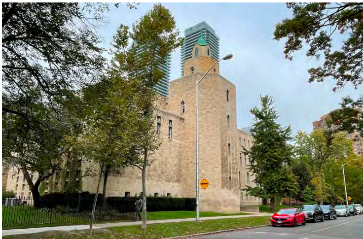
24. Carr Hall, 1950-54, 100 St. Joseph Street, Ernest Cormier with Brennan & Whale architects (HP, 2021)
