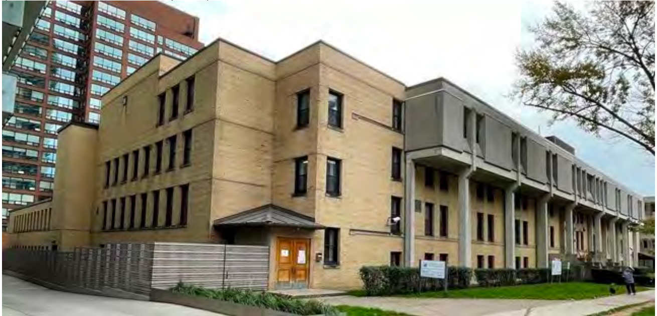
38. St. Basil's Seminary, side (east) and principal (north) facades with later additions including the two-storey extension (far left), 4th floor extension on the north elevation and the new single storey entrance. (HP, 2021)
