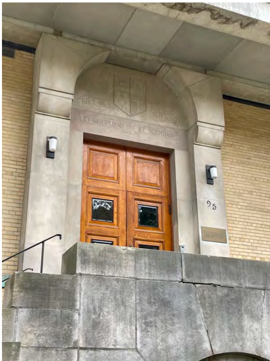
45. Principal Entry on the north elevation (HP, 2020)
