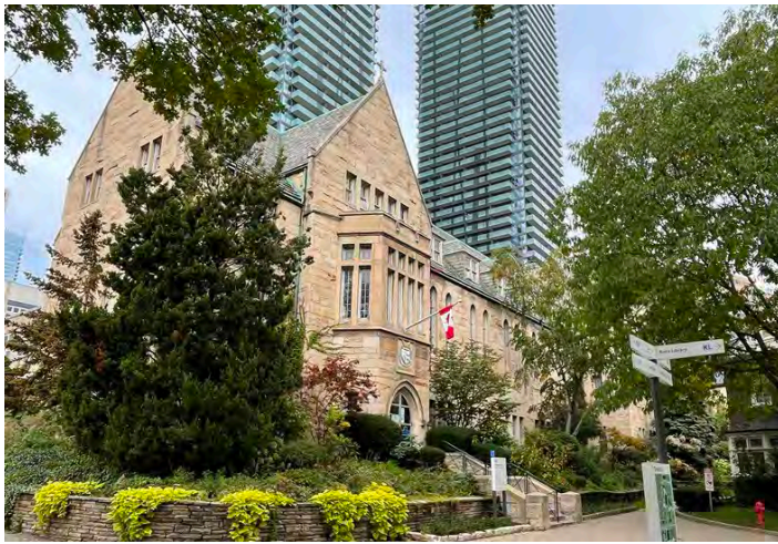
20. Brennan Hall, 1937, west and south elevations, A. W. Holmes. (HP, 2021)
