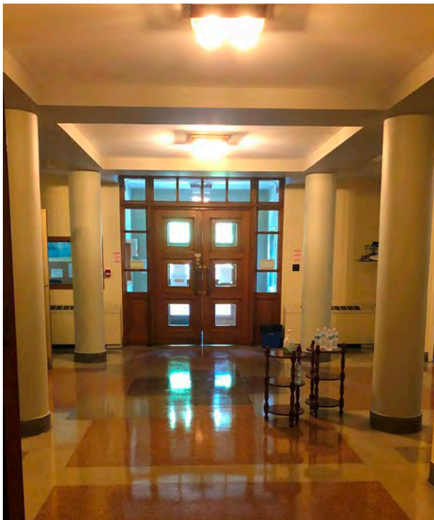
58. Interior of the main lobby with the intersection of the two corridors marked with a cruciform plan, four columns and terrazzo patterning in the floors (HP, 2020)
