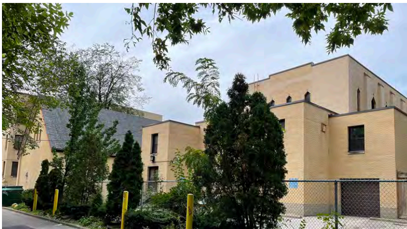
49. View of the south and east elevations of Newman Chapel (far left) and the seminary chapel, sacristy and ancillary spaces facing St. Basil Lane looking west. (HP, 2021)
