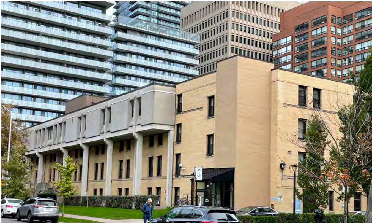
39. St. Basil's Seminary, principal (north) façade and side (west) façade with later stair tower and glazed entrance at the corner. (HP, 2021)
