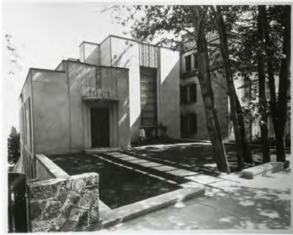
31. Photograph of the principle façade of the Cormier House, Montreal, 1930-31, designed by Ernest Cormier. (Ernest Cormier fonds, Canadian Centre for Architecture)
