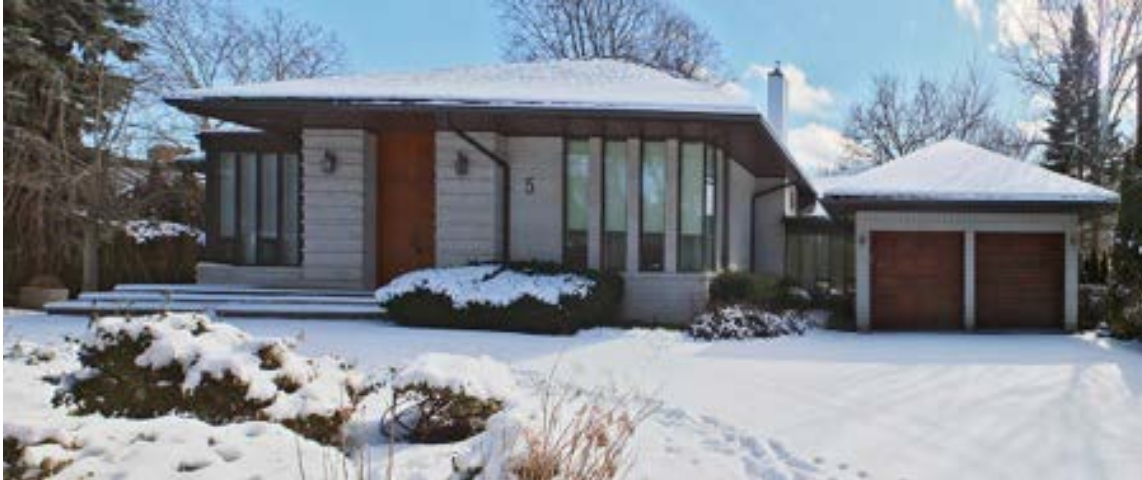
5 Dale Avenue- north view of house from Dale Avenue
