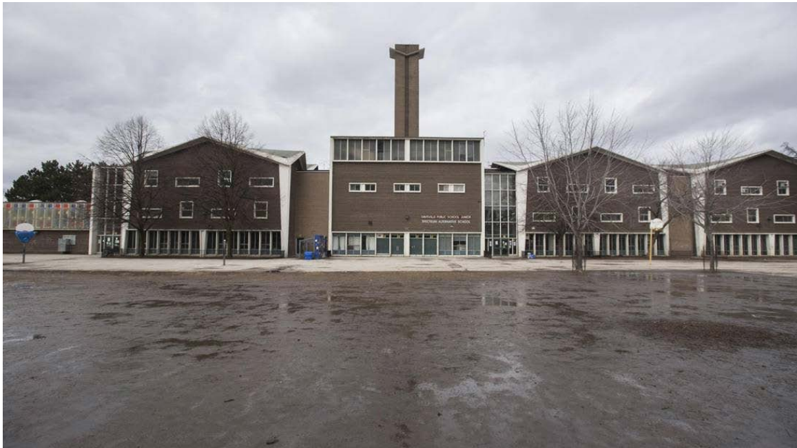
The structure which houses both Davisville Junior Public School and Spectrum Alternative Senior School will be replaced by a new building right next door. Fred Lum/The Globe and Mail
