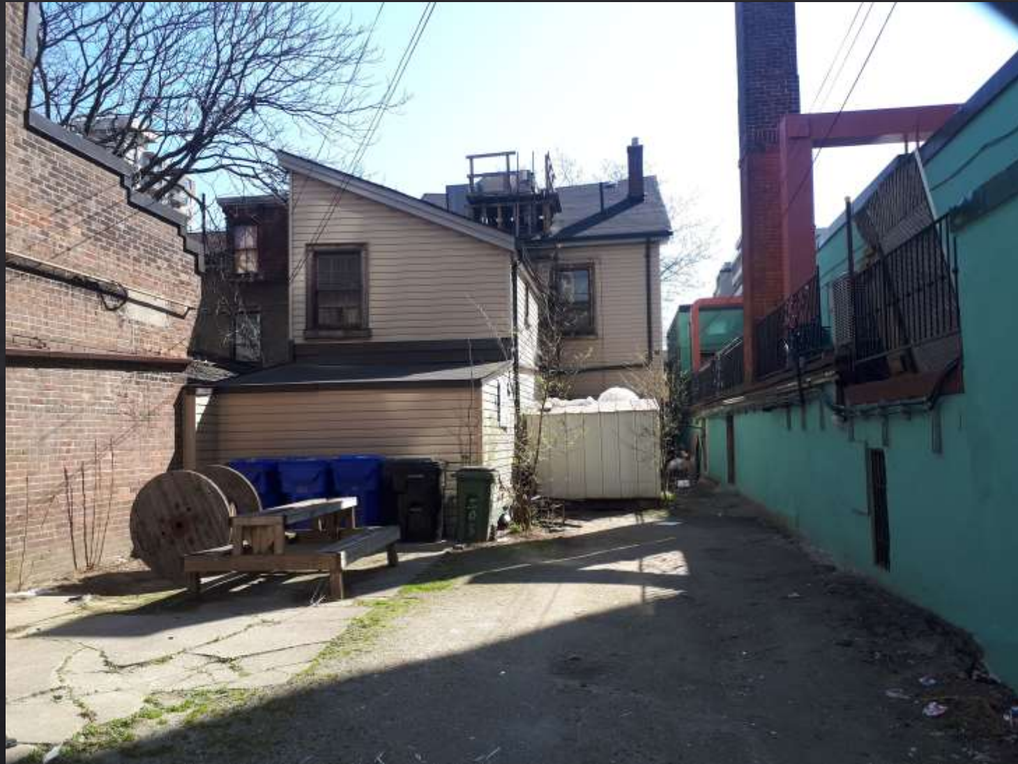
The Rear (West Elevation) of 506 Church Street, Toronto: 3 May 2020.
