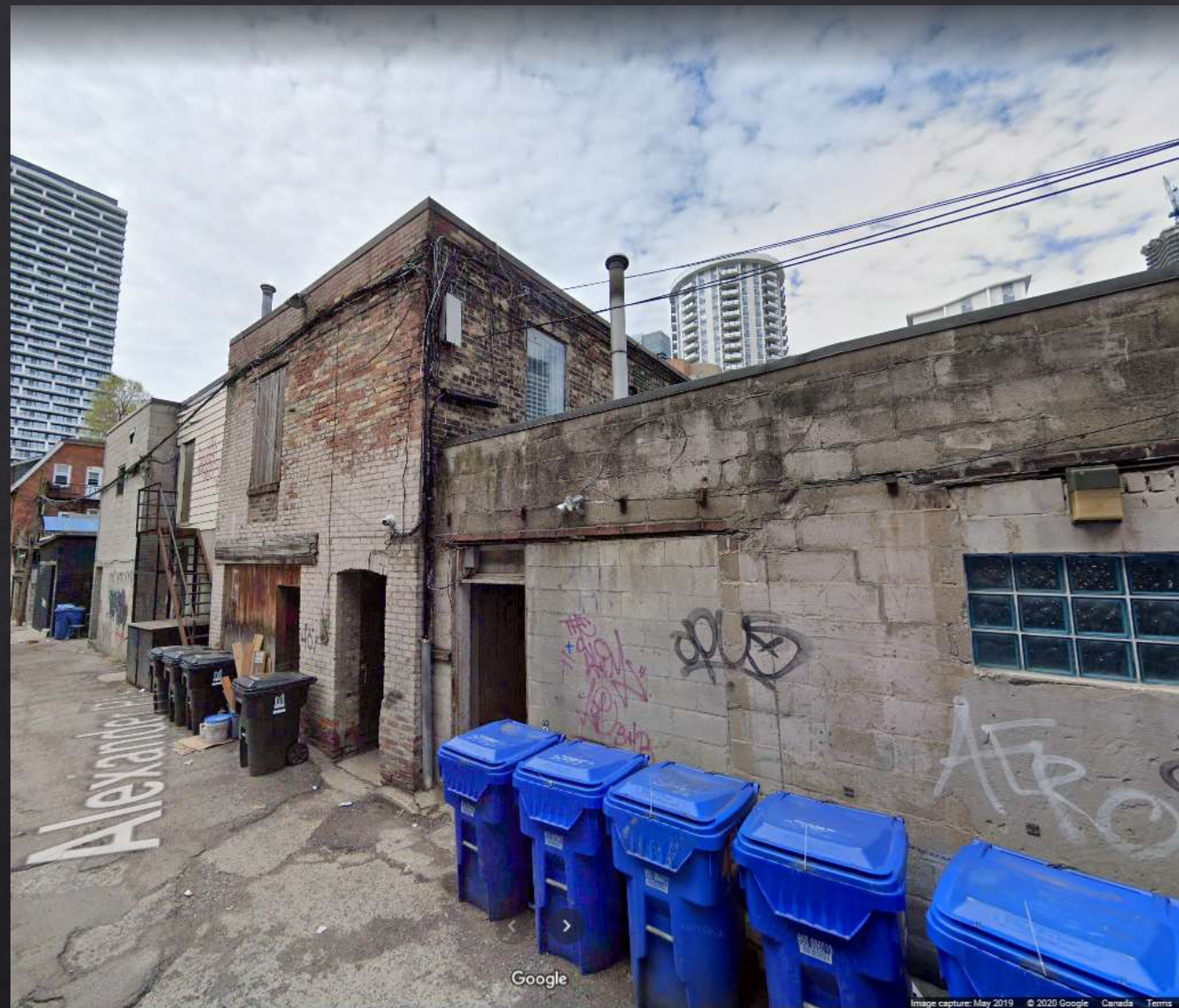
East (Alexander Place / Rear Laneway) Elevation of 467-471 Church Street, Toronto.
