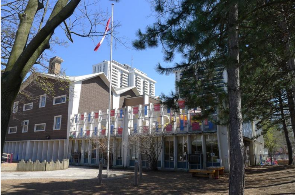
25. Day Nursery Wing : showing the roof top playground at the second level with colourful panels on the enclosure. The Junior School is at the left of the photograph. (HPS, 2016)
