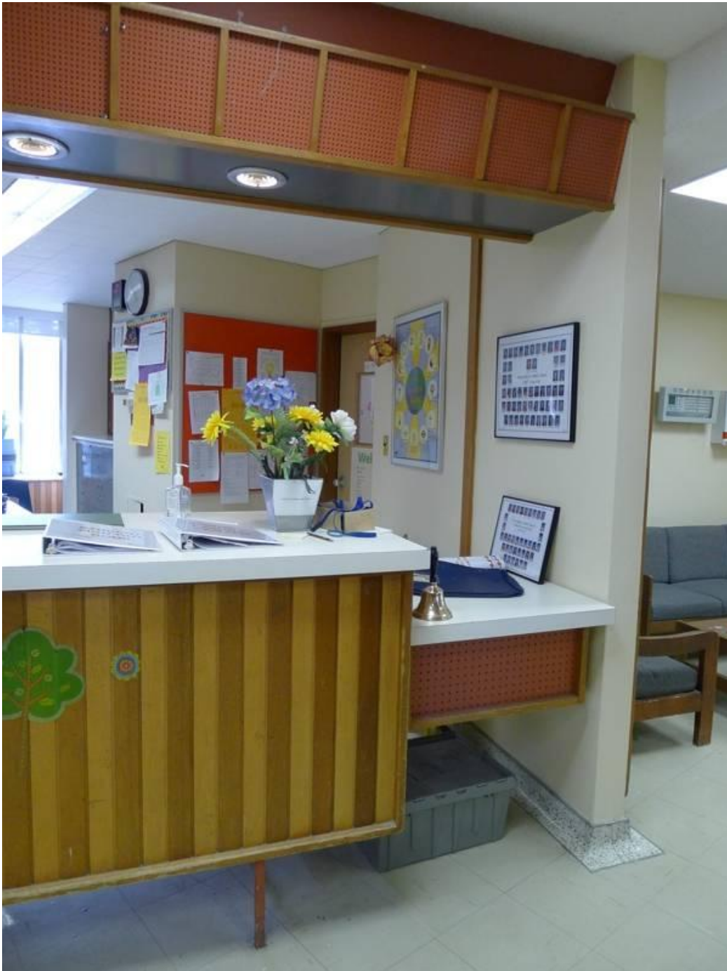
38. Entry Lobby Counter : showing the details with the lower level counter for the children with the red perforated masonite, the two-tone striped desk, the original lighting with the red masonite and soffit in blue (HPS, 2016)
