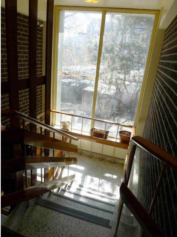
46. Day Nursery Staircase : showing the stairs which are built into the walls and the multiple handrails for additional safety. (HPS, 2016)
