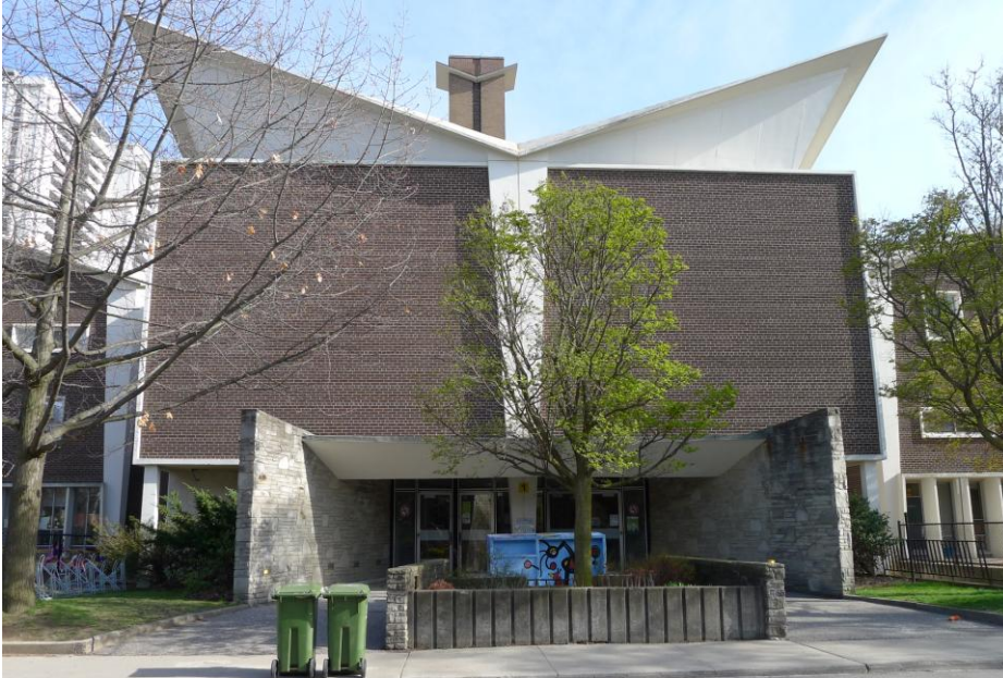
29. Entry Pavilion, North Elevation facing Millwood Road : showing the dramatic roof, the stone walls supporting the inverted canopy, extending forward, and the low stone walls around the original planting area for the tree and the adjacent school wings. Note the chimney with its parallel inverted decorative concrete element. (HPS, 2016)
