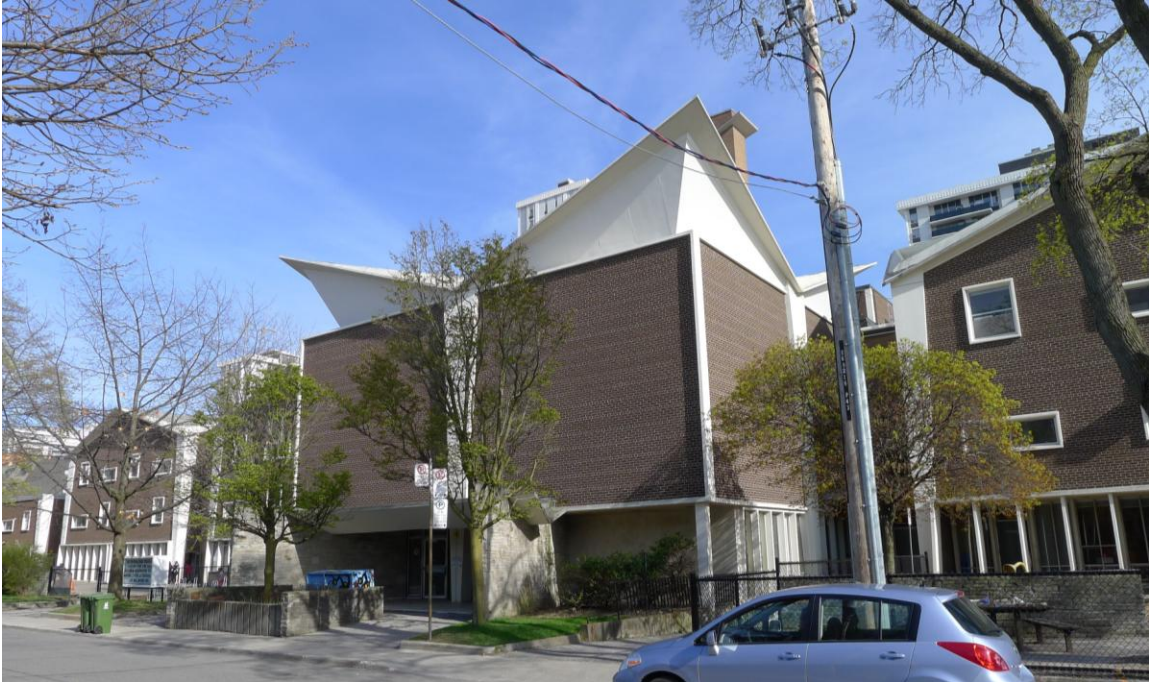
15. North Elevation of the Metropolitan Toronto School for the Deaf and the Davisville Junior School, 1962 facing Millwood Road: showing the central entry pavilion with its dramatic four-corner inverted roof, the Junior School on the right and the School for the Deaf at the left. (HPS, May 2016)
