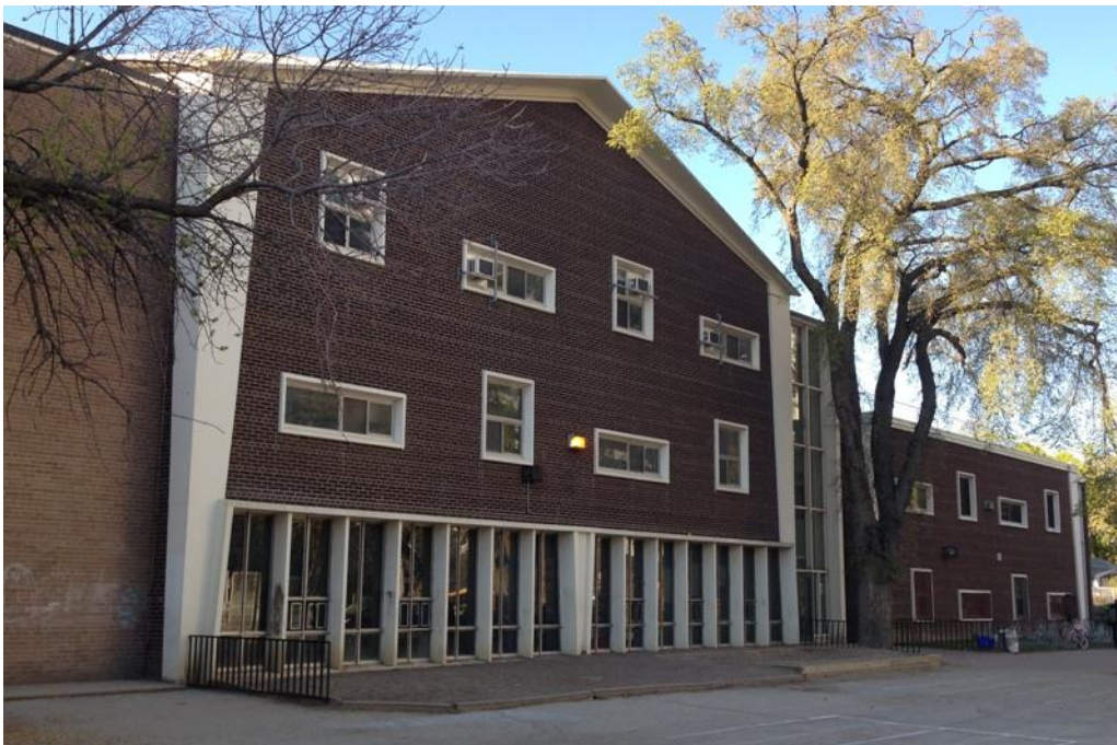
28. South Elevation with 1965-6 Addition (far right) : showing one of the original School for the Deaf pavilions with the linking elements which are either in the lighter, buff brick cladding or fully-glazed staircase elements, and at the far right the 1965-6 addition which lacks the gable-roof form, the parabolic roof and is set on the ground without the 'colonnade' of full-height windows. (HPS, 2016)
