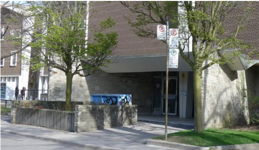
30. The Main School Entrance facing Millwood Road : showing the planter with the field-stone and concrete walls around the tree planter and the field-stone walls supporting the inverted concrete canopy which extends beyond the stone walls. (HPS, 2016)
