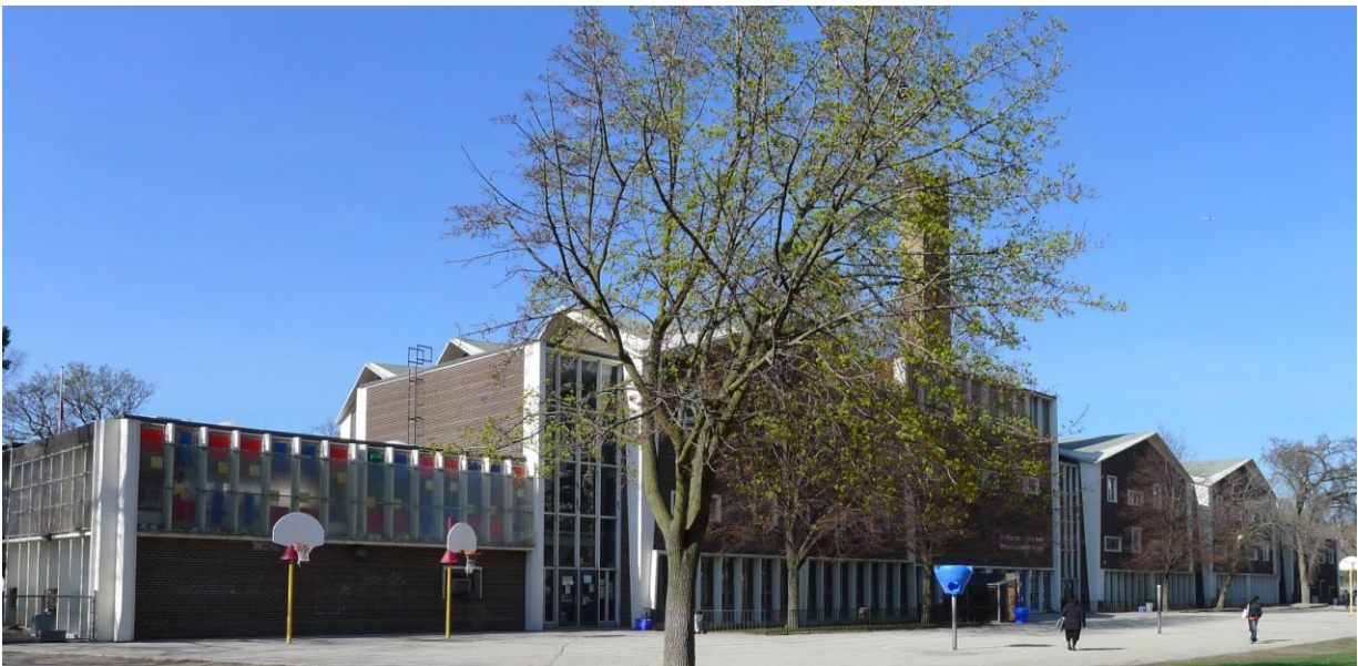
22. South Elevation of the School facing the Playground : showing the day nursery with roof top playground, on the left, and the assembly of pavilions with linking elements enclosing stairs or other services in between. (HPS, 2016)
