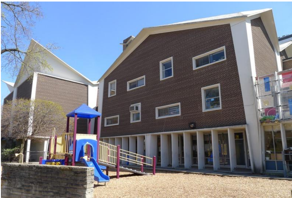
20. Junior School Wing, North Elevation : showing entry pavilion at the left and the house-like form of the pavilion, with first floor 'colonnade' of pre-cast concrete fins and full-length windows extending to the ground providing visual continuity with the playground and the playful arrangement of the windows at the second and third floor levels. In the foreground is an original stone playground wall. ( HPS, 2016 )
