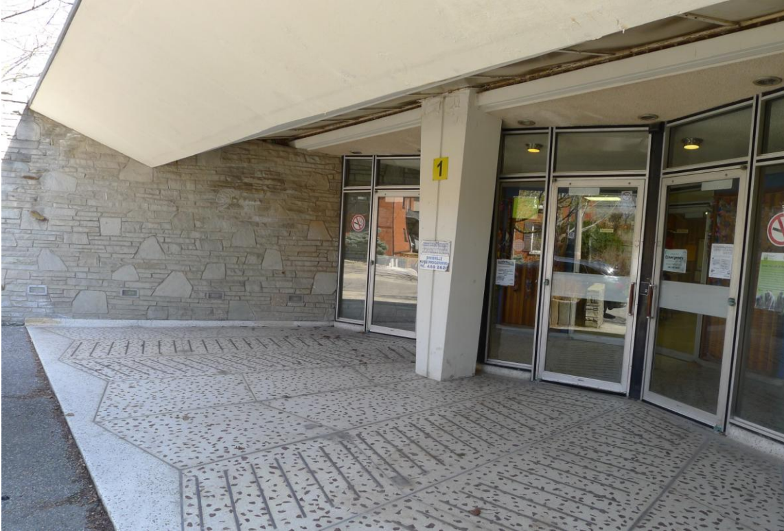
32. The Main School Entrance : showing the inverted concrete canopy, the pier separating the two entrances for the two schools, the zig-zag pattern of the doors with the corresponding zig-zag patterns in the terrazzo and one of two field stone walls framing the entrance with the various sized stones. (HPS, 2016)
