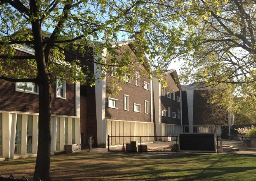
21. School for the Deaf, North Elevation : showing the 1965-6 addition on the left with the two pavilions for the School for the Deaf in the centre and the projecting entry pavilion at the right. As at the junior school the ground floor colonnades of thin concrete fins and full-length windows provide continuity with the exterior and a more domestic scale is maintained at the upper floors. (HPS, 2016)
