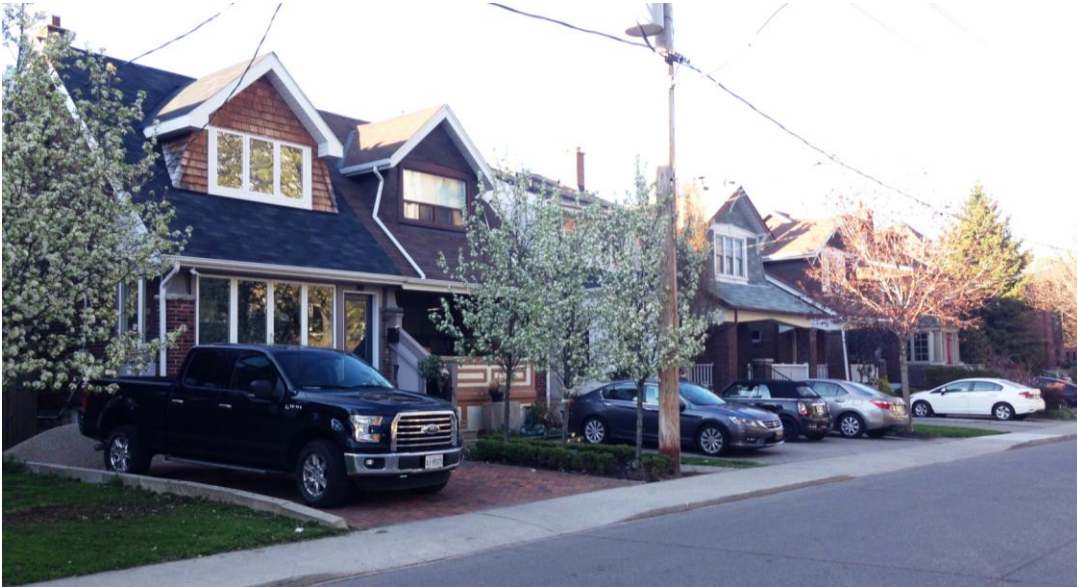
48. North side of Millwood Road : showing additional residential context of Millwood Road facing the school. (HPS, 2016)
