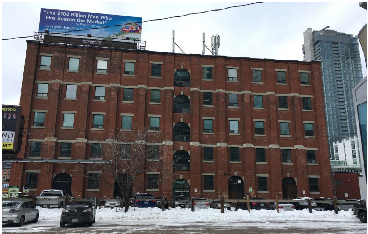
View of the south facade of the Steele Briggs Building (ERA Architects)
