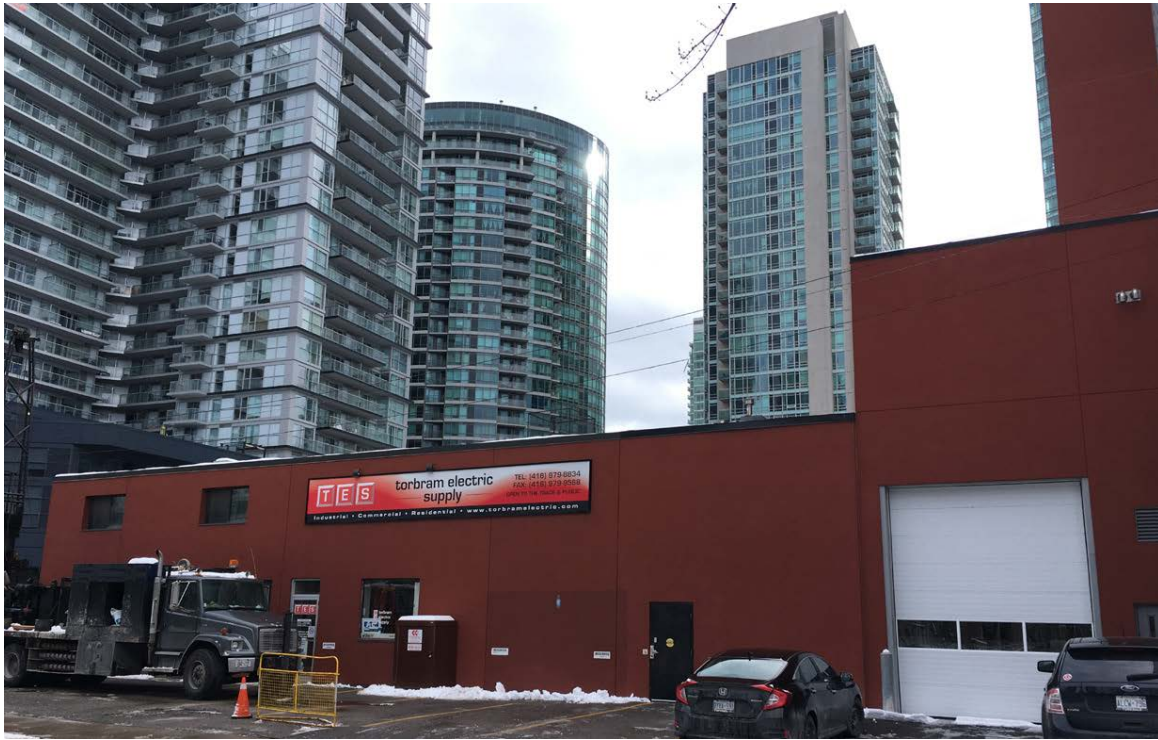
View of the north wall of the low scale addition on the eastern edge of the Steele Briggs Building (ERA Architects)
