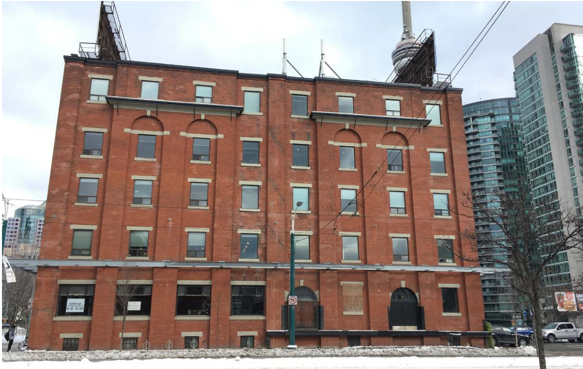
View of the west (Spadina Avenue) facade of the Steele Briggs Building (ERA Architects)
