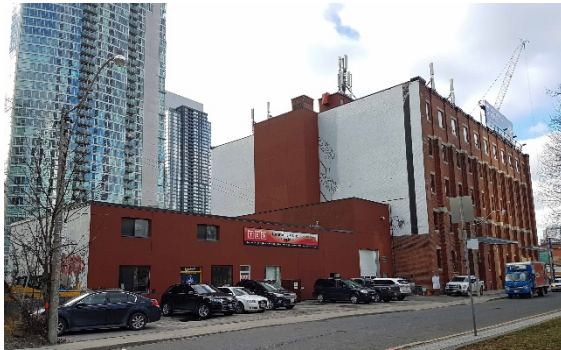
5d. east elevation and wing
