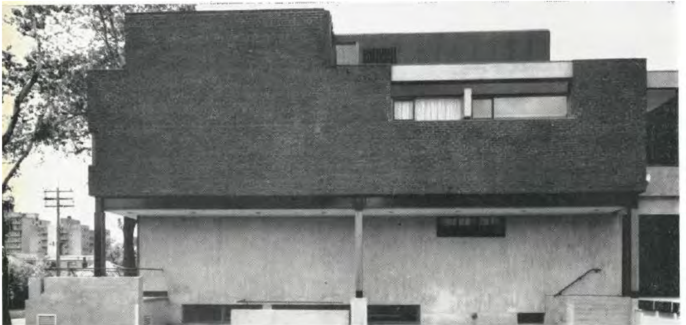
67. Photograph of the East elevation and loading dock, showing the restroom and washroom windows of the second floor, kitchen window of the first floor and basement windows, with curtain wall of the office section to the right ( Canadian Architect , September 1962, p. 46)
