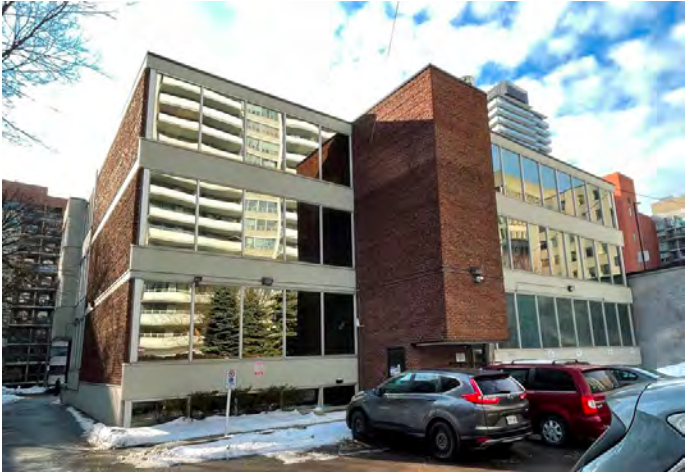
71. North and east elevations showing the rear, north side with the projecting, brick-clad volume of the staircase and third floor addition completed in 1970 (HP, 2022)
