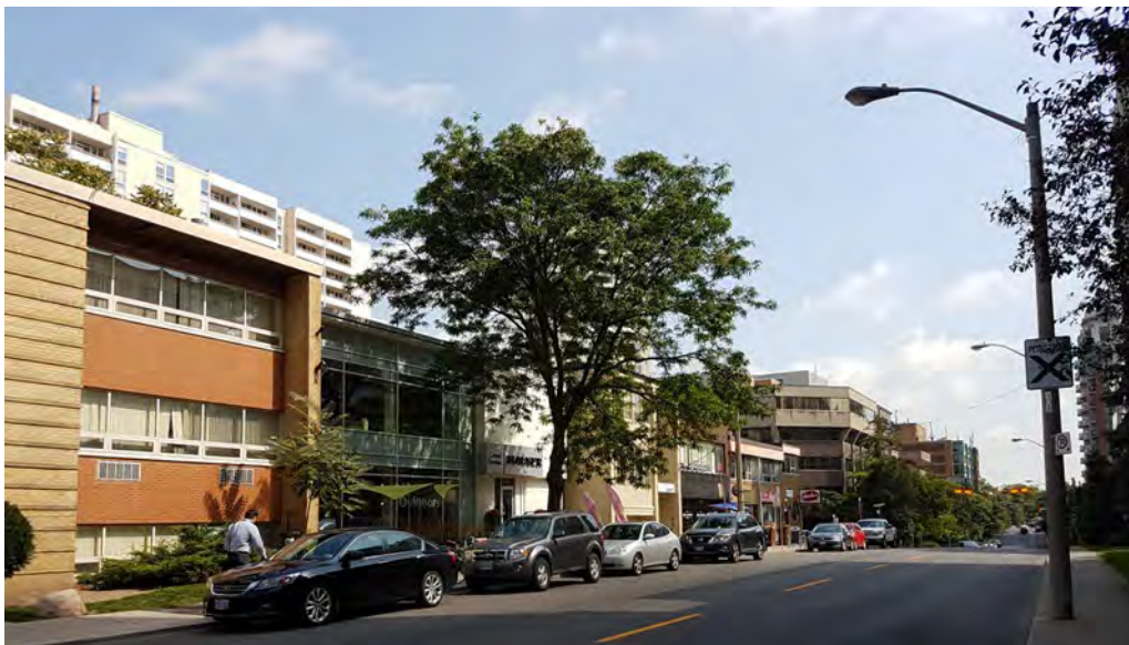
107. East end of Merton Street towards Pailton Crescent showing the examples of low-rise commercial buildings. (HP, 2017)
