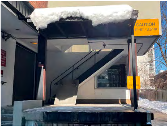
69. East side with loading dock and 1970-72 fire escape stairs (HP, 2022)
