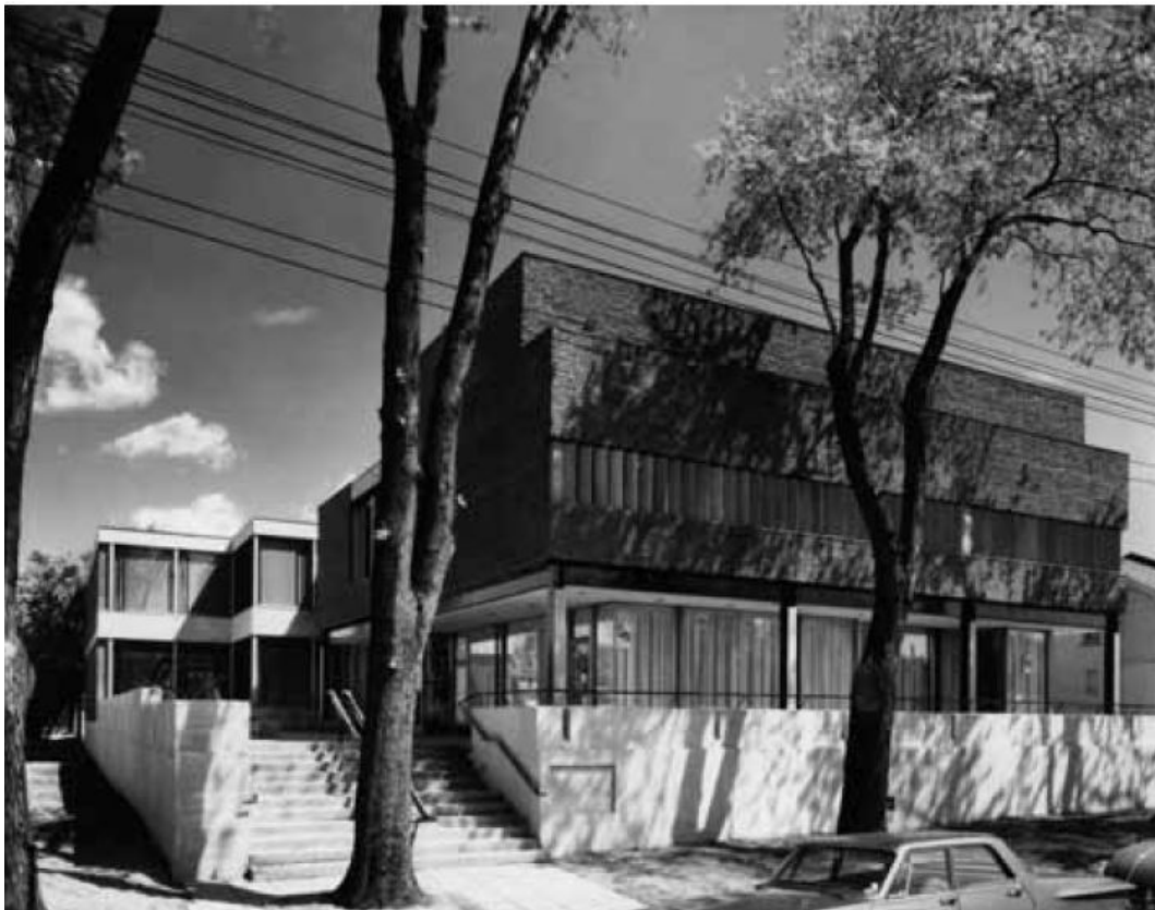
39. Girl Guides of Canada Headquarters, shortly after completion in 1962 (Baird, 2016, p. 41)
