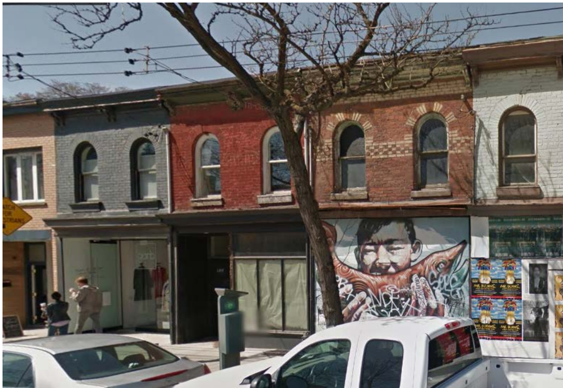
1042, 1044 and 1046 Queen Street West (from right to left) (Google Maps 2015)
