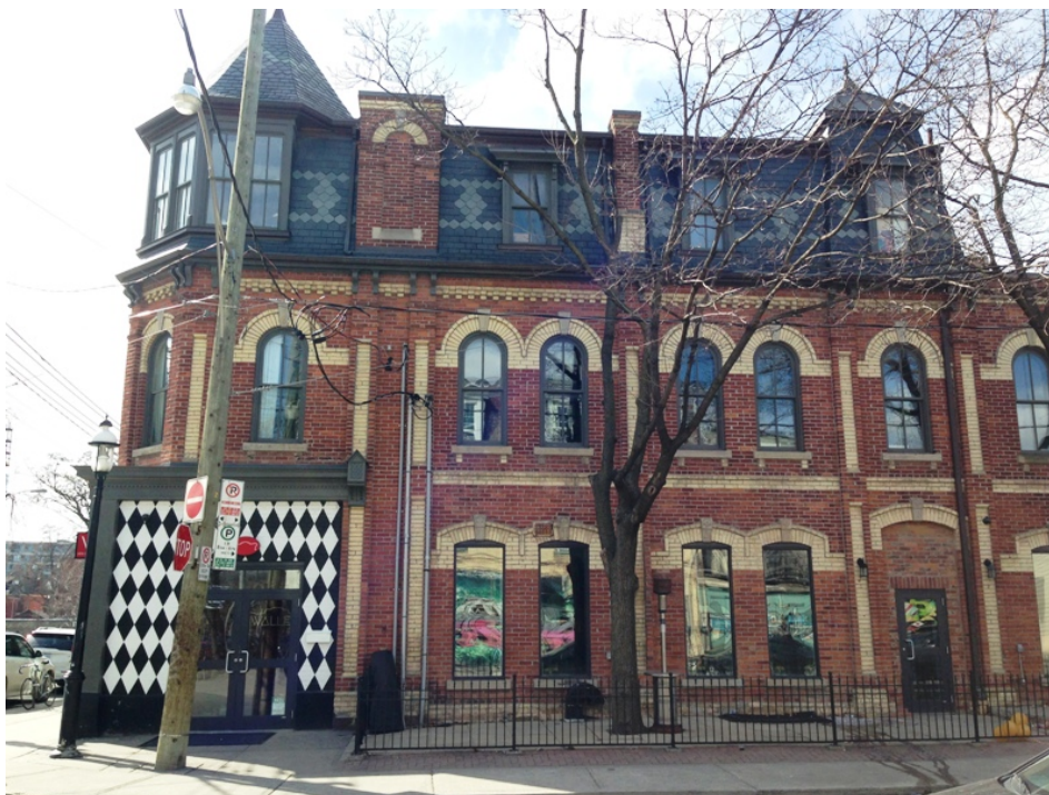
9. Vogan Block, east elevation, front, three-storey portion (HPS, 2017)
