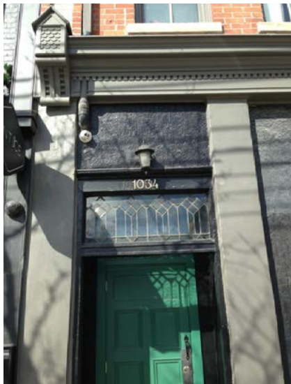
14. Vogan Block, South Elevation, entrance to 1034 Queen Street West showing the corbel bracket and wood cornice and the leaded transom light above the door.
