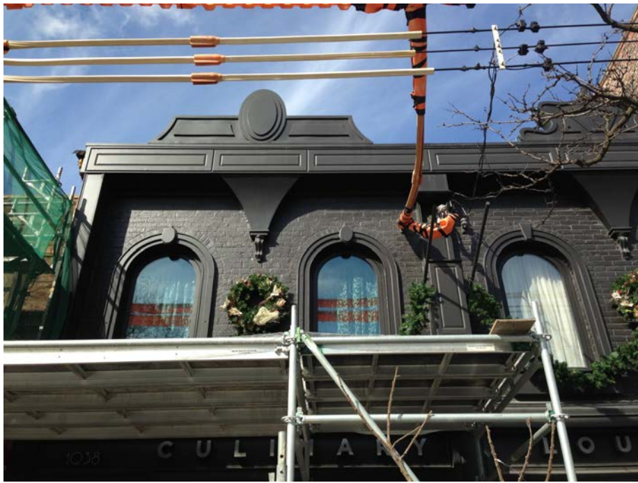
18. 1036-1038 Queen Street West: showing recent additions including the cornice and parapet as well as the mouldings around the windows at the second floor (HPS, 2017)
