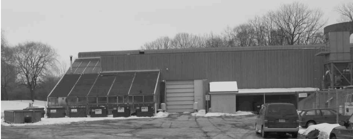
Greenhouse addition and access area to workshop areas – Valley Building C
