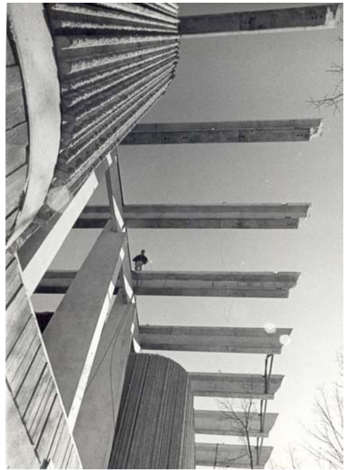
Precast concrete structure under construction
