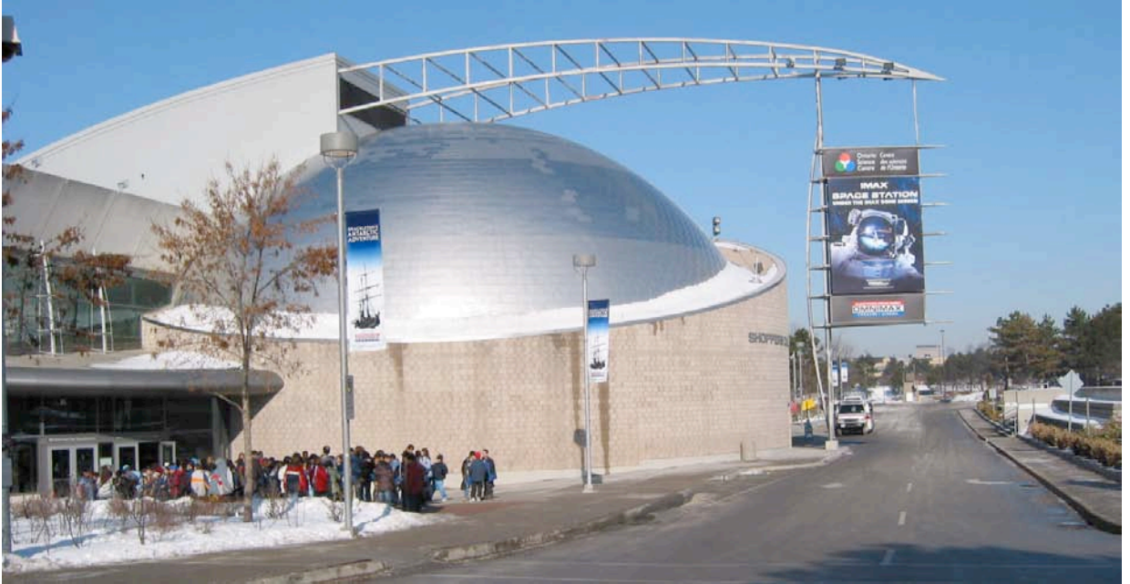
Group Entrance – Lower Level Building A
