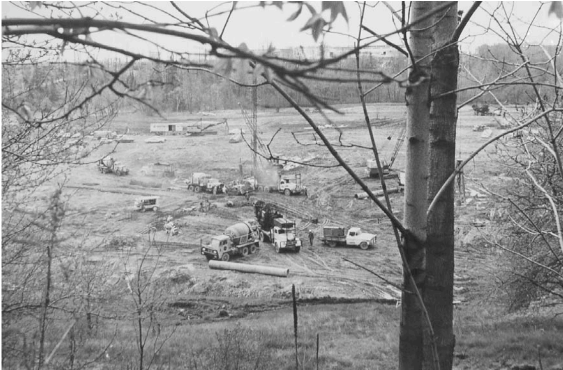
2.9 Valley Building C – Foundations Construction, late May, 1966
