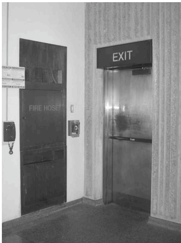
Fire hose/waste receptacle and bronze exit sign and door
