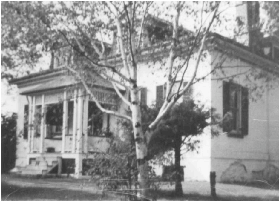
2.2 Meagher House on OSC site (demolished 1965) See also section E-4.2
