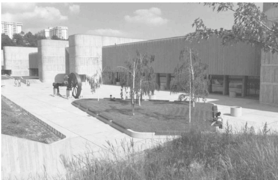
2.7 Original North Patio, Valley Building
