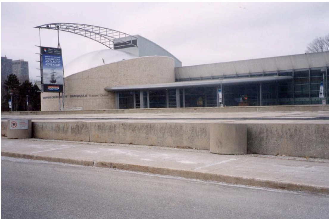
Plate 2: Looking southeast to fountain and main Science Centre reception building.
