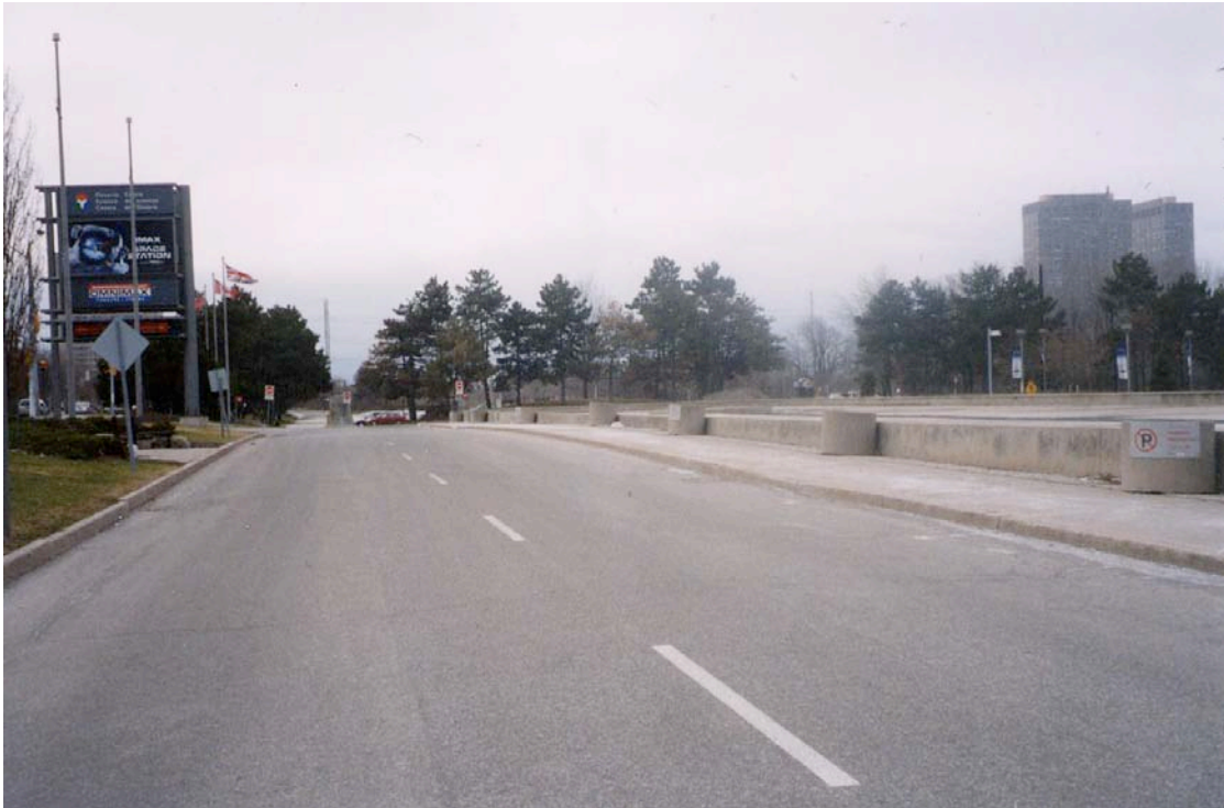
Plate 1: Looking south along eastern boundary of study area. Landscaped berm parallel to Don Mills, interior road and fountain within Science Centre complex are visible.
