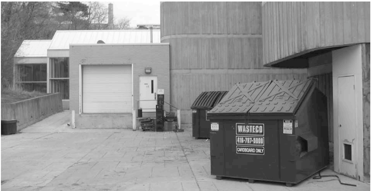
Service area to restaurant addition in patio area in valley adjacent to Building C
