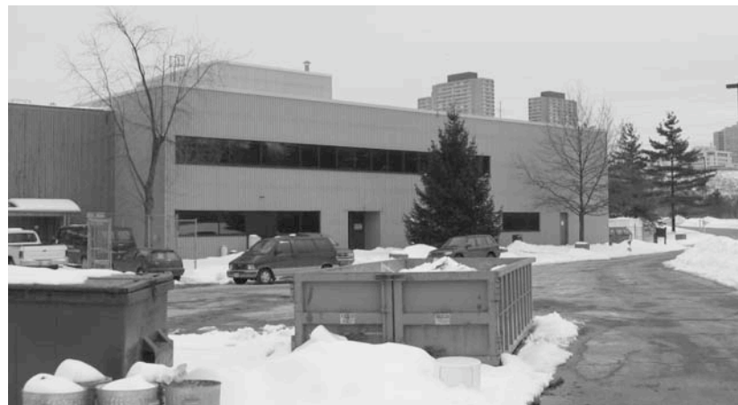
West façade of storage and Workshop Addition – Building C
