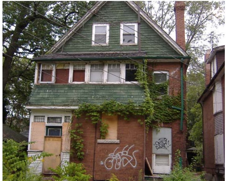
↑ One of the houses approved by the OMB for demolition.
