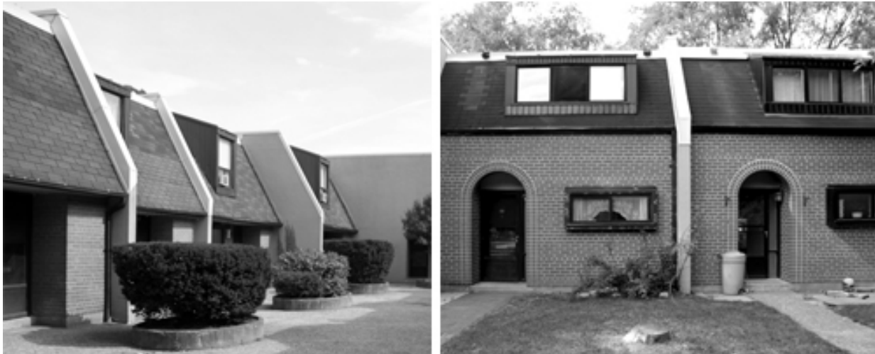
Figure 37: Don Valley Woods, photo undated (Source: E.R.A. Architects 1967).
