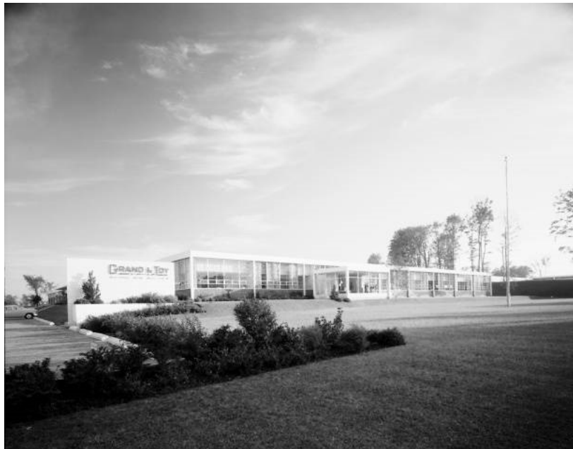
Figure 19: View of 33 Green Belt Drive, 1958, showing expansive lawns, hedged borders, treed areas close to buildings, and conveniently located parking areas. (Source: Canadian Architectural Archives, Libraries & Cultural Resources, University of Calgary, Image No. 55203-6).
