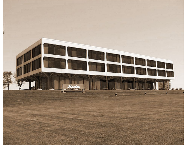
Figure 29: Headquarters of the Bata Shoe Organization exhibiting International Style and landscape, 2013 (Source: Bata Brands SA, Wikimedia Commons).
