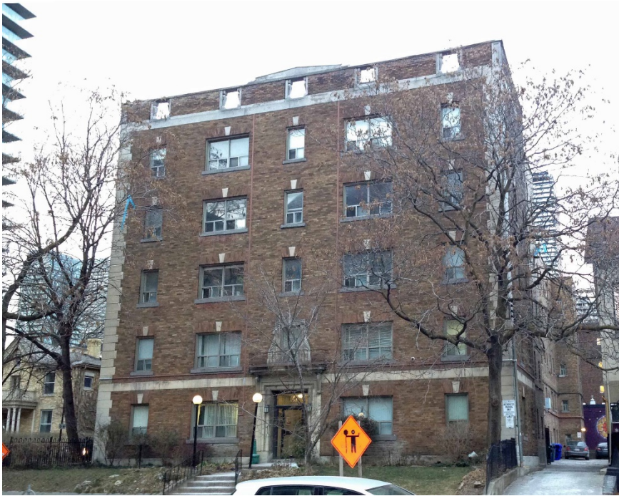
4a. principal (south) elevation (left) and east side elevation (right)
