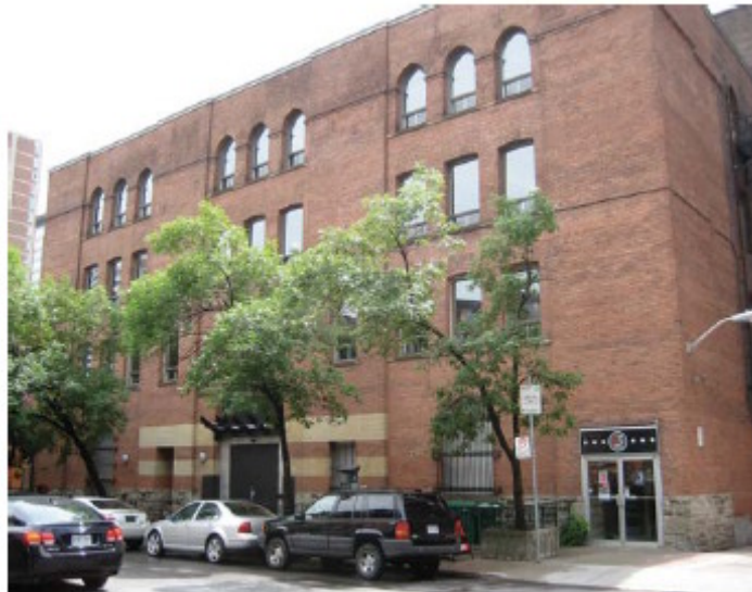
Figure 10: North facade of 5-9 St. Joseph Street. Source: ERA.
