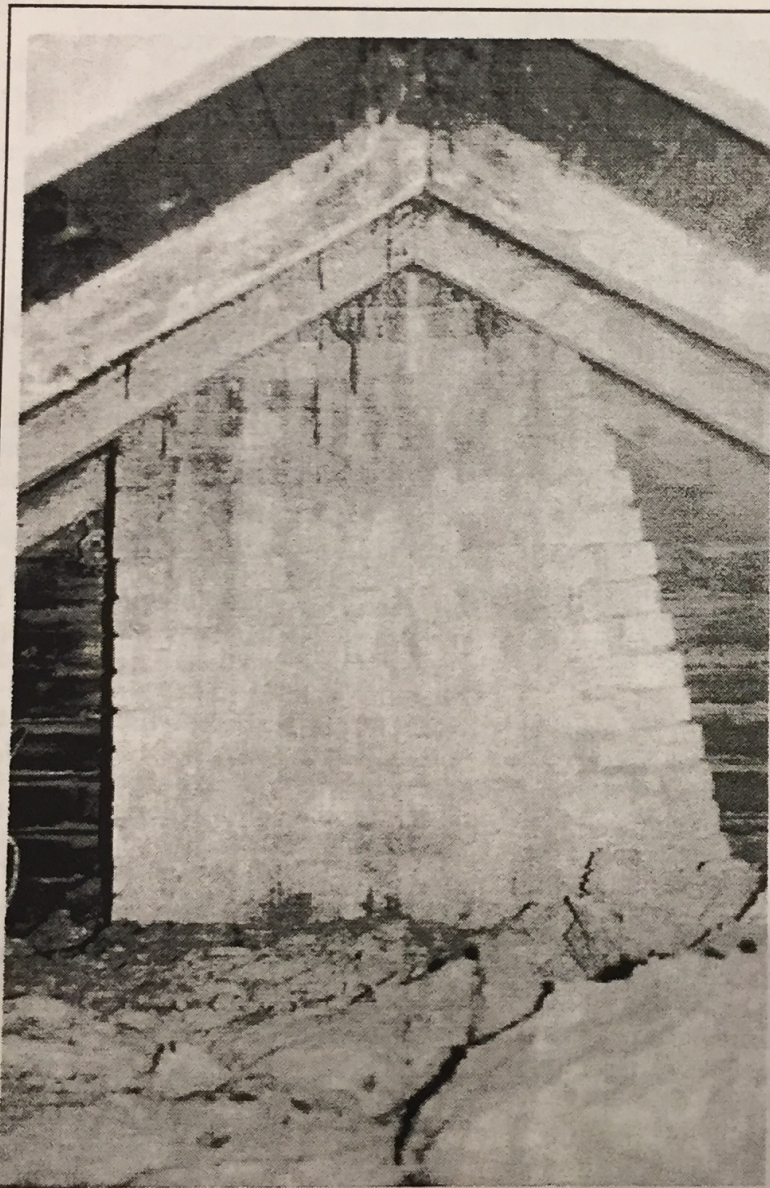
Illustration 4. Photograph of upper chimney in loft.
