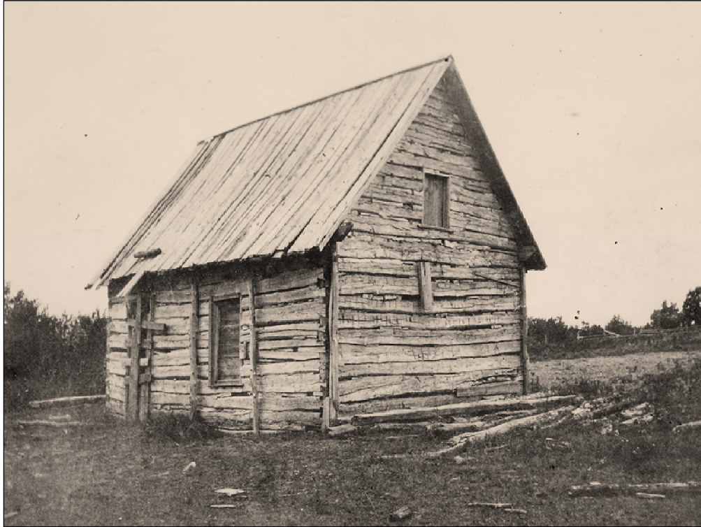
Figure 9 Reverend Roddick log house, SE 17-9-18W, ca. 1900. This dovetail-joined log house was dismantled in the 1950s. (Murray McPherson.)
