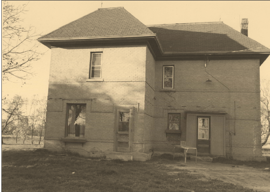
Figure 29 Cristine House, SW 17-11-19W, ca. 1890. The exclusion of a verandah that was originally planned for this house provides an unobstructed view of the interesting brick detailing.
