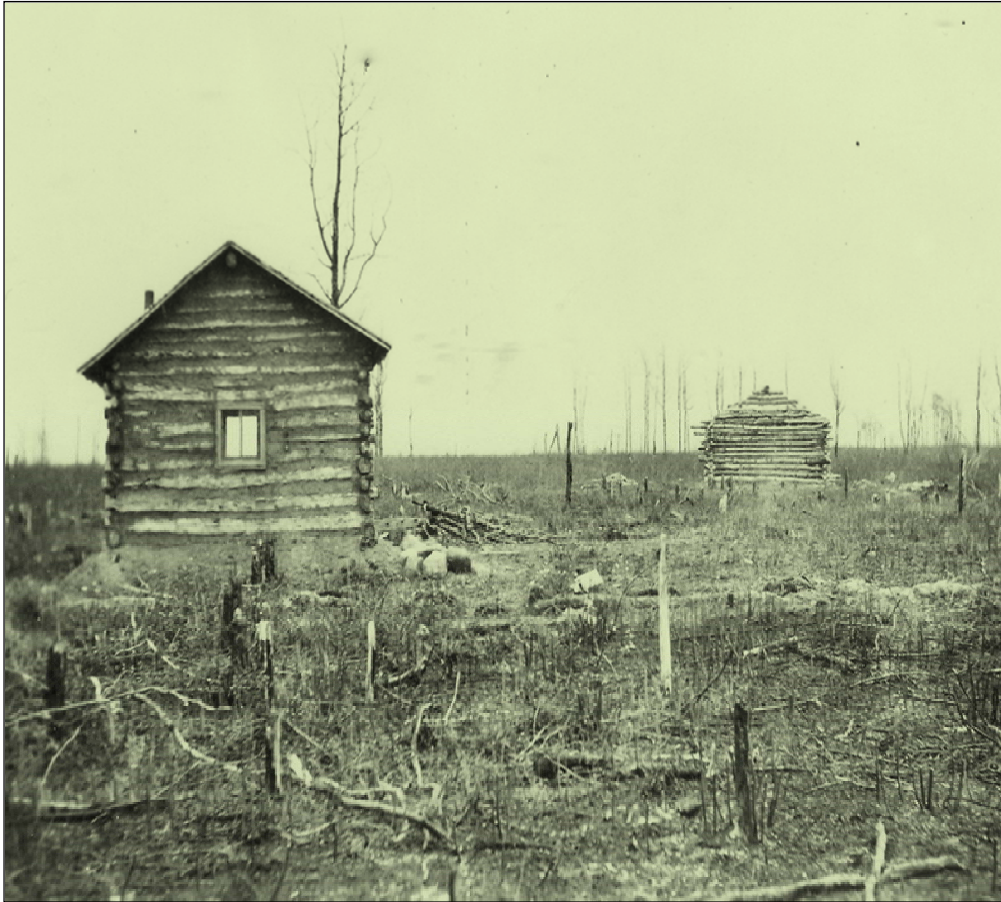
Figure 8 Reverend Roddick log cabin, SE 17-9-18W, ca. 1879. This house was probably one of the first built in the planning district, and this image suggests the rough pioneer experience. (Murray McPherson.)
