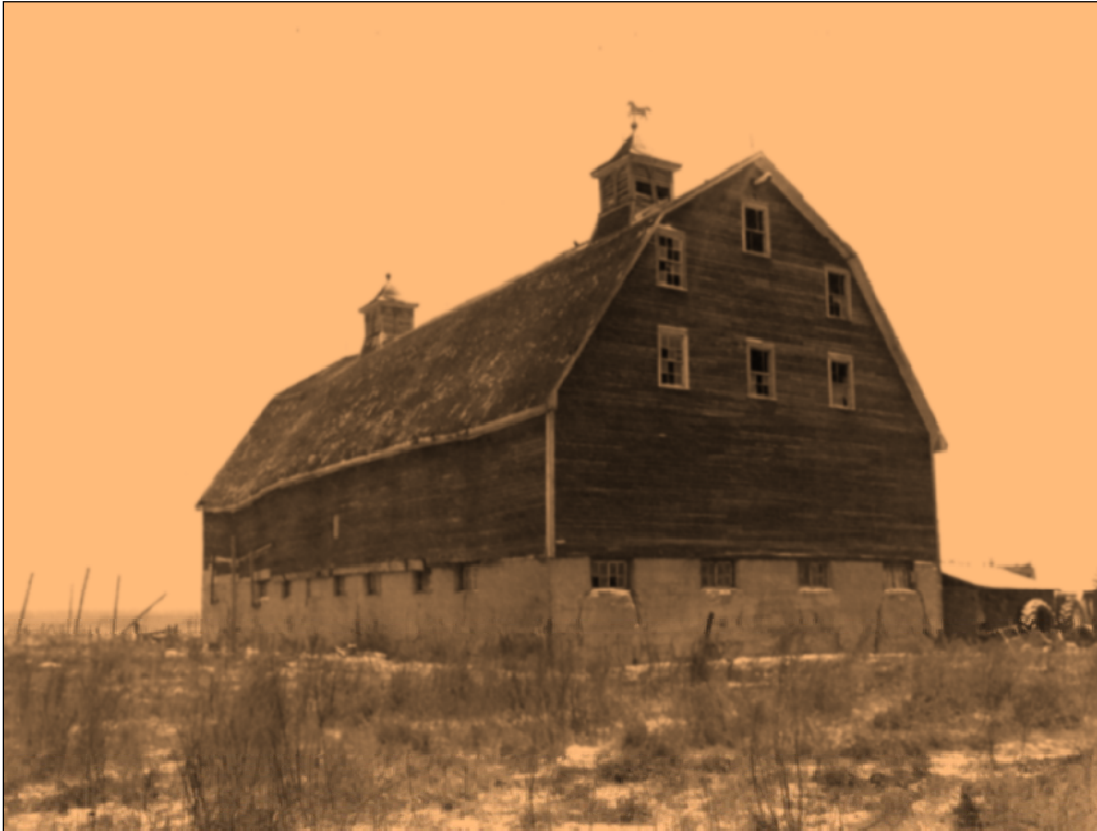
Figure 56 Shields Barn, NW 18-9-19W, 1910-12: southeast view.
