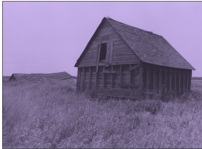
Figure 61 Granary, NW 13-9-10W. The hatch in the gable end was used for loading and unloading the grain. Bags of grain were usually pitched from a wagon up to the opening.
