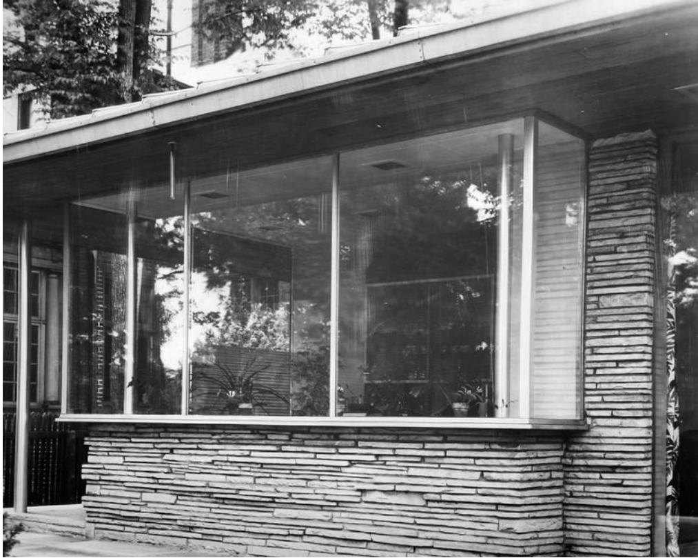
Non-glass walls were constructed of a buff flagstone. GORDON S. ADAMSON & ASSOCIATES
