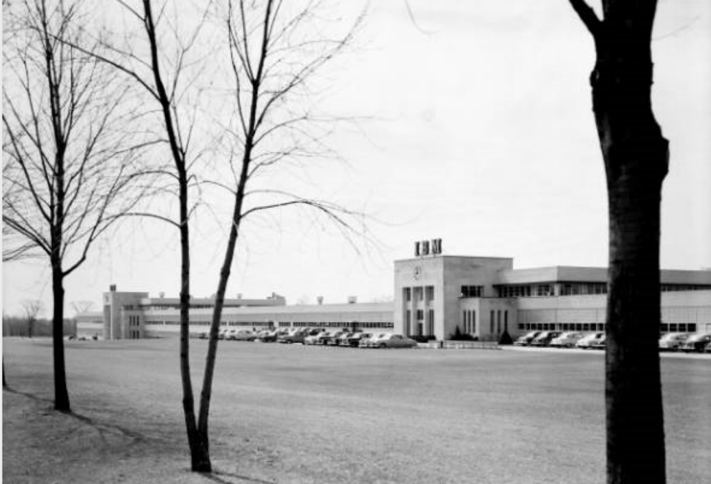
20. View from Don Mills Road looking south at the IBM Head Office and Factory: showing the dramatic extent of the building, which now includes the 1954 extension and its deep set back from Don Mills Road with a broad lanscape of lawns and a line of trees parallel to the road. (Canadian Architectural Archives(CAA), Panda,54416-4_2 )
