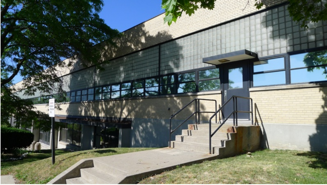
28. IBM/Celestica, East Elevation : showing the same entrance as the image above with replacement handrails. (HPS, 2016)
