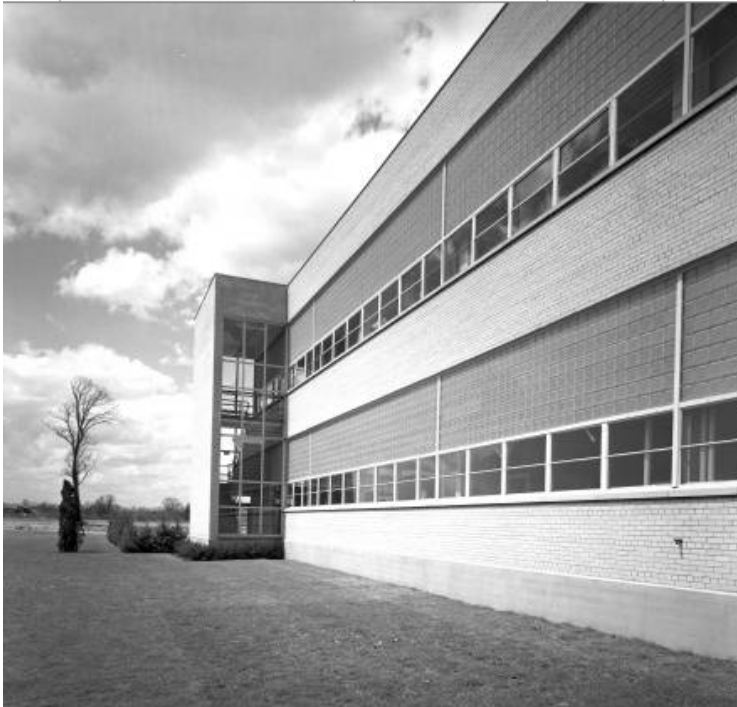
30. IBM, South Elevation : showing the transparent effects of the projecting staircase on the 1954 extension and the vast farmland landscape beyond to the west. (CAA, Panda, 54436-18)
