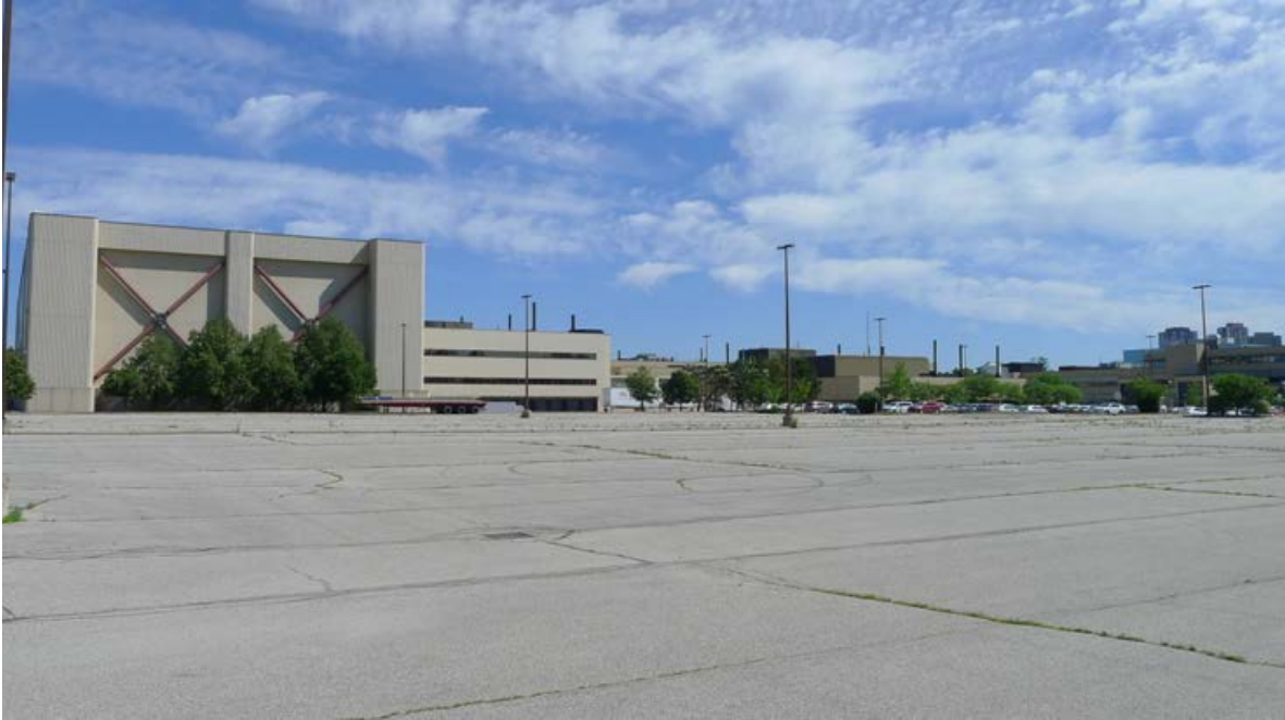
17. IBM/Celestica : looking north-east from the parking lot near Eglinton Avenue, showing the 1980 extensions on the left and those of 1970 at the centre with the original IBM complex at the far right ( HPS, 2016 )
