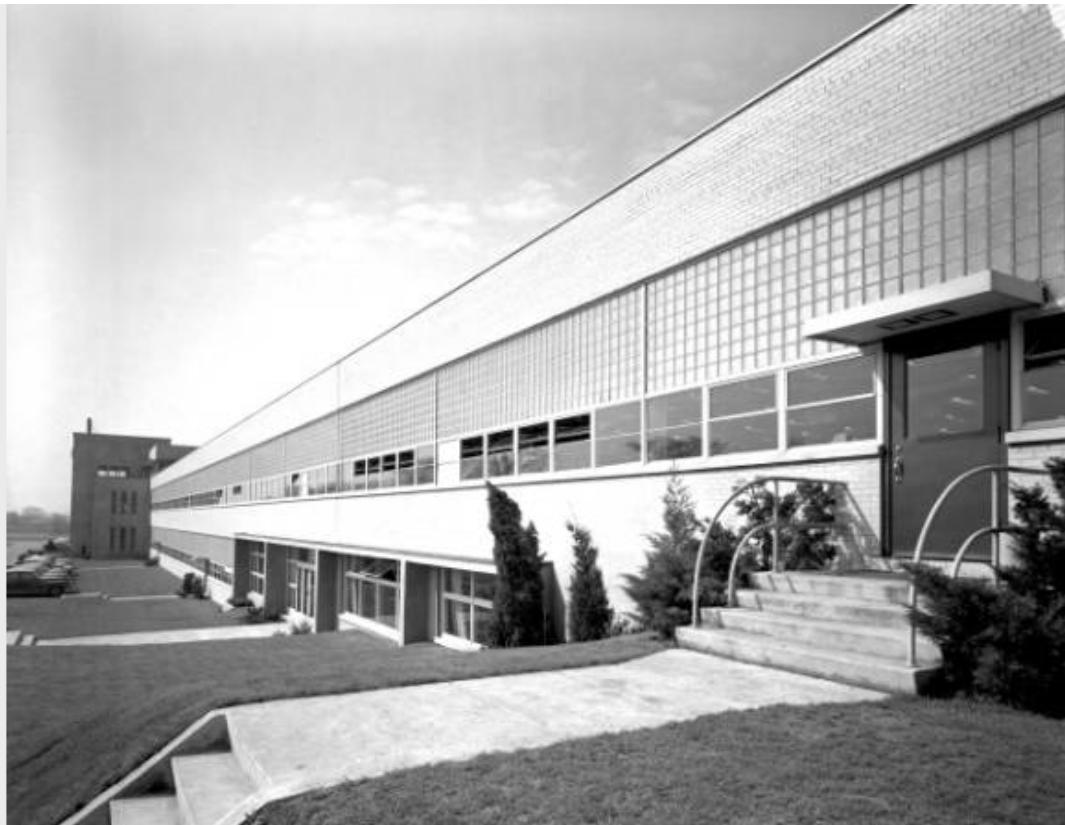
27. IBM Building, East Elevation : showing one of the minor entries on the 1951 portion of the building with its projecting canopy and handrails. (CAA, Panda,54416-2)
