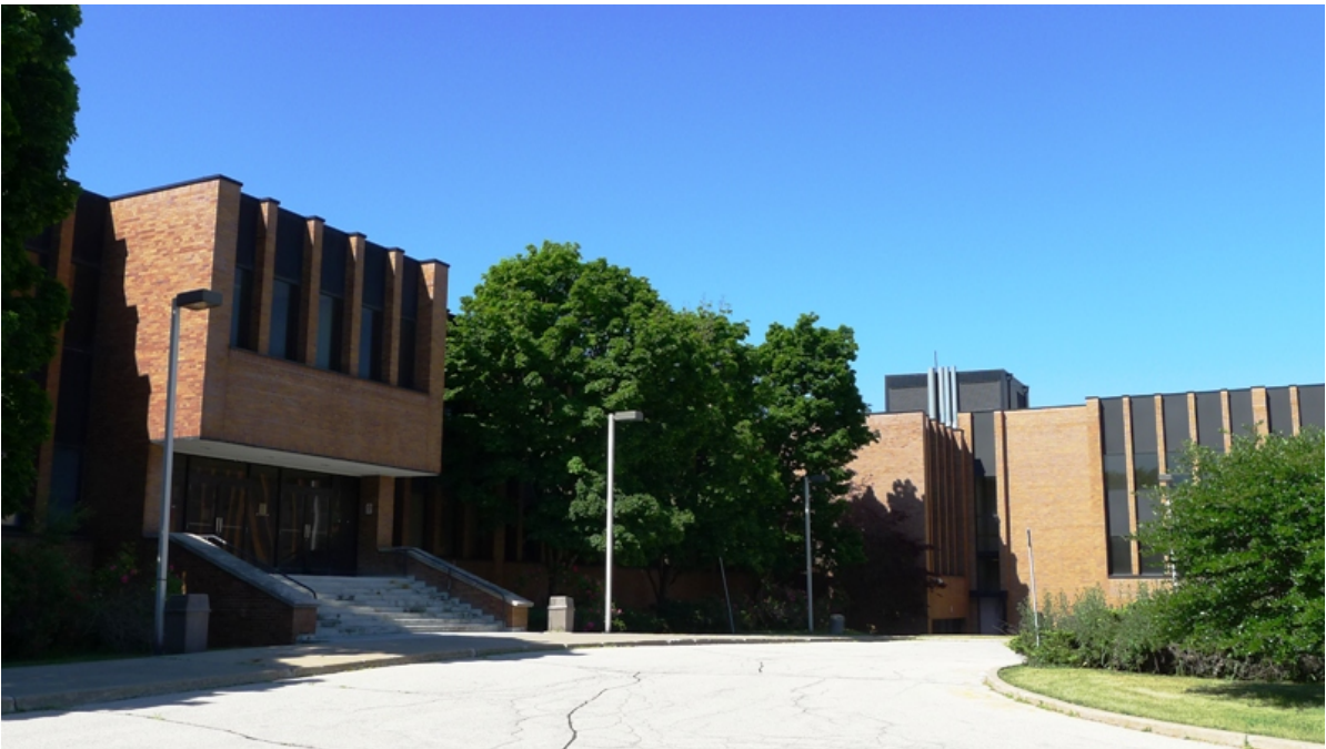
42. North Courtyard with Main Entry : showing the entry forecourt planting and wide steps leading up to the main entry with a bay cantilevered over the recessed doors (HPS, 2016)
