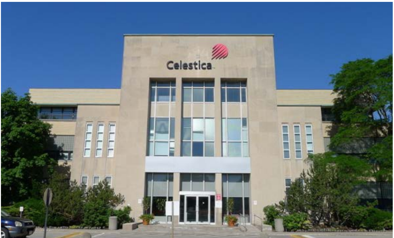
25. IBM/Celestica, south entry pavilion : showing the 1954 south entry pavilion with a three-storey central bay flanked by two-storey side bays all clad in stone and featuring vertical windows. ( HPS, 2016 )
