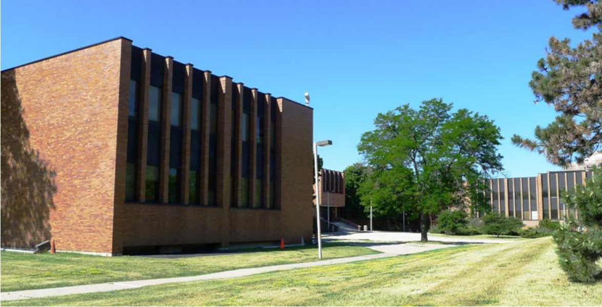
39. IBM Headquarters, 1966-7 : looking west at the north elevations and the northwards facing entry court with various plantings ( HPS, 2016 )
