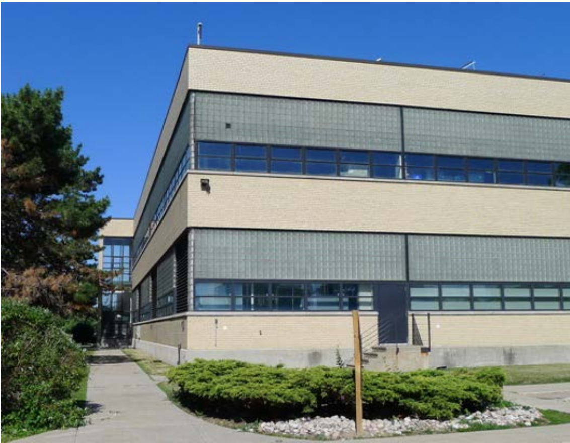
29. IBM/Celestica, East Elevation : showing the south wing completed in 1954, with later entrance and handrail details. (HPS, 2016)
