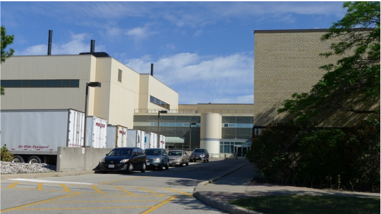
18. IBM/Celestica : showing an additional view of the 1970 extensions to 844 Don Mills Road by NORR ( HPS, 2016 )
