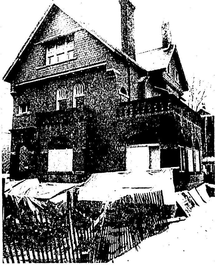
The old house on Spadina Road which is slated to become a subway station.
