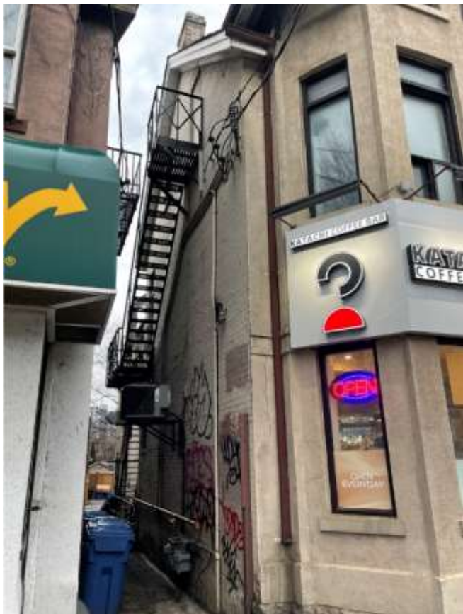
Figure 23: Side (east) elevation of 199 College Street, as viewed from College Street (Heritage Planning, 2022).
