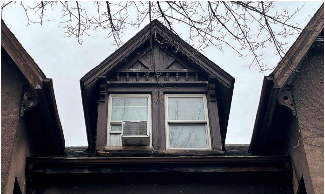
Figure 20: Dormer woodwork detail, 193-195 College Street (Heritage Planning, 2022).
