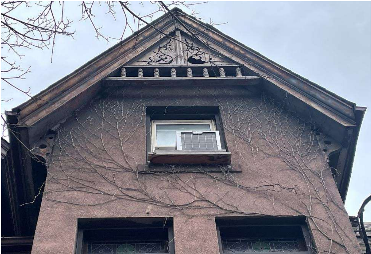
Figure 19: Gable woodwork detail, 195 College Street (Heritage Planning, 2022).
