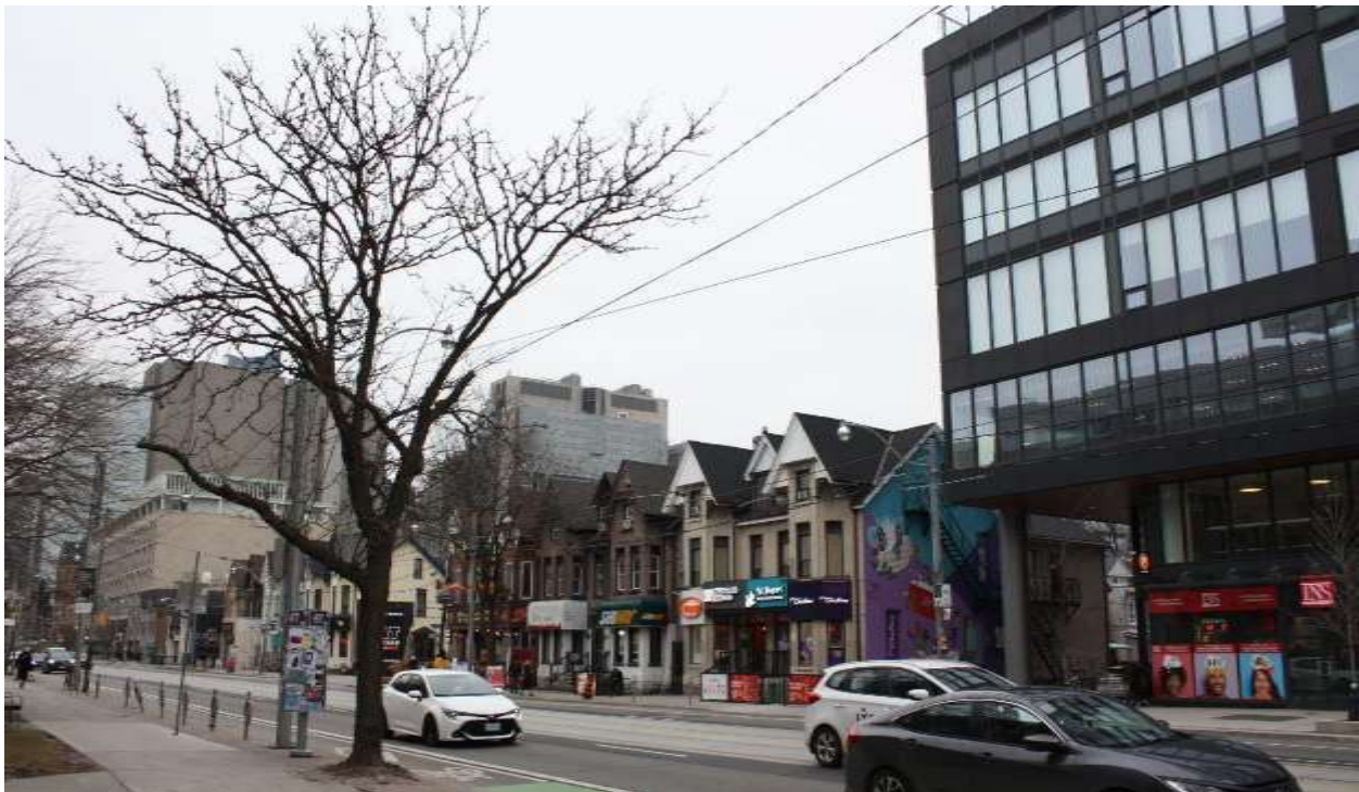
Figure 30: View of 191-199 College Street from the northwest (Heritage Planning, 2023).
