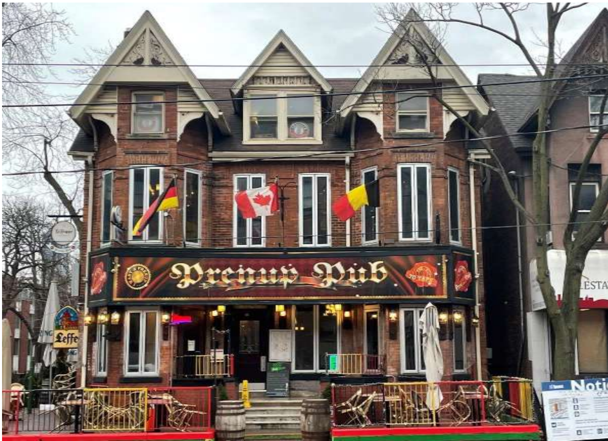
Figure 11: Principal (north) elevation of 191 College Street (Heritage Planning, 2022).
