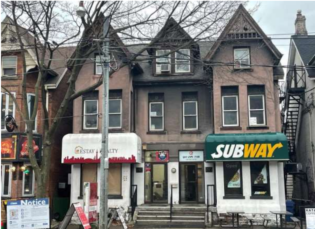
Figure 16: Principal (north) elevations of 193-195 College Street (Heritage Planning, 2022).
