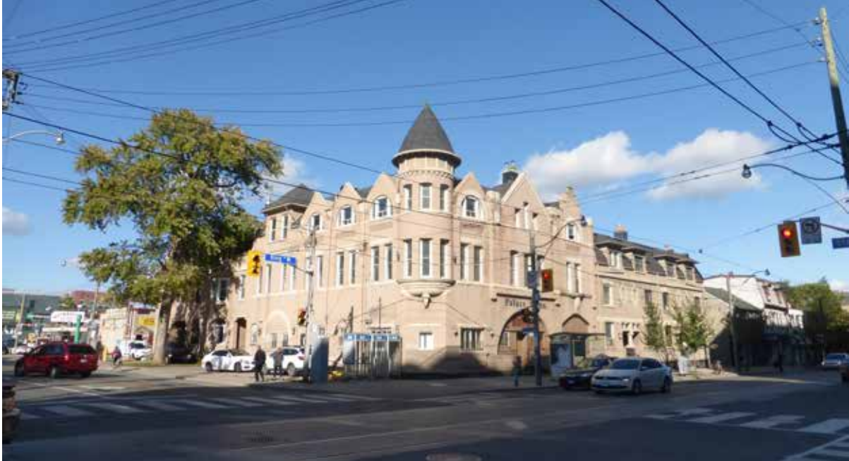
Looking north-east on King Street West (ERA, 2017).
