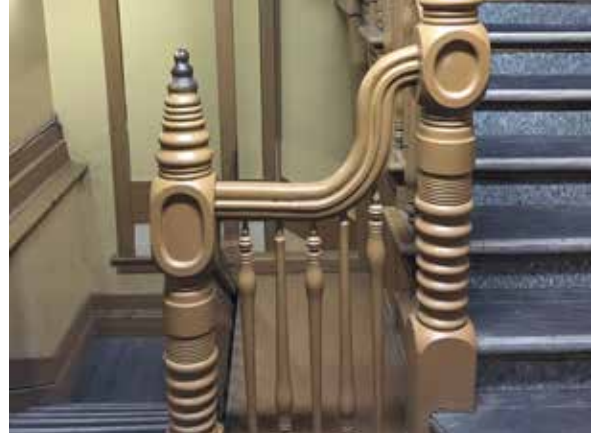
Staircase decorative elements in good condition, 950 King St. W. (ERA, 2017)
