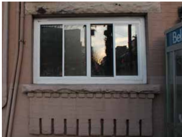
Modern replacement window unit in fair condition (ERA, 2017)
