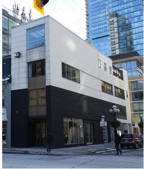
35. 878 Yonge Street (Source: ERA Architects)
