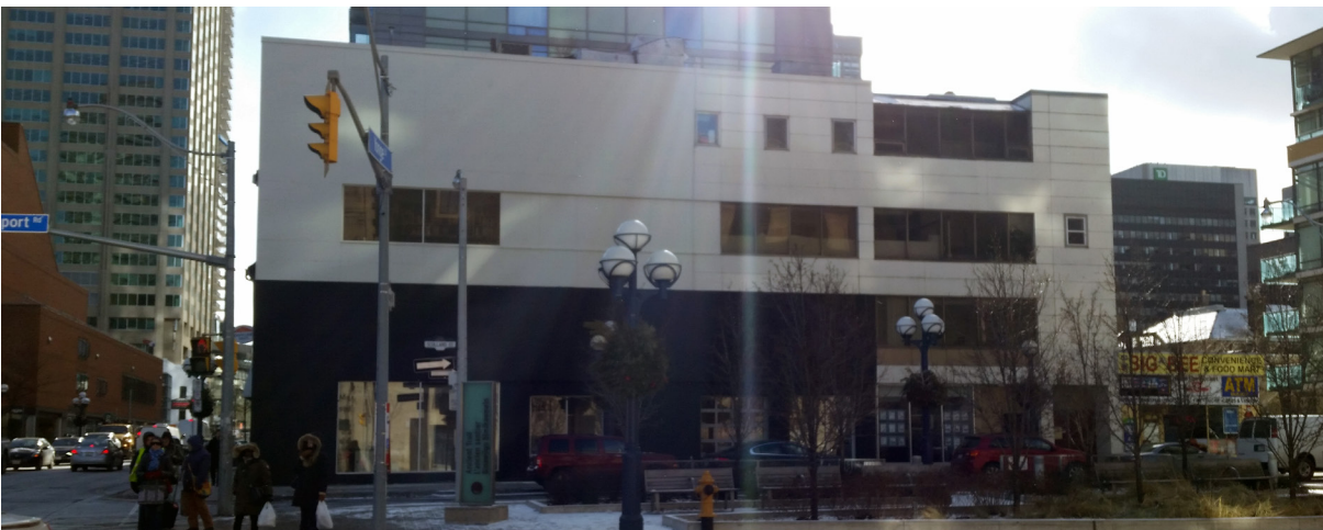
36. 878 Yonge Street (Source: ERA Architects)
