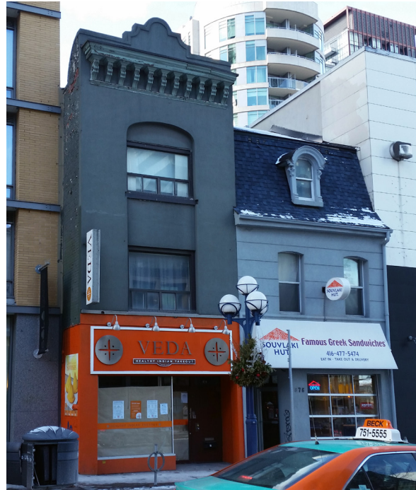
18. 874 & 876 Yonge Street (Source: ERA Architects)
