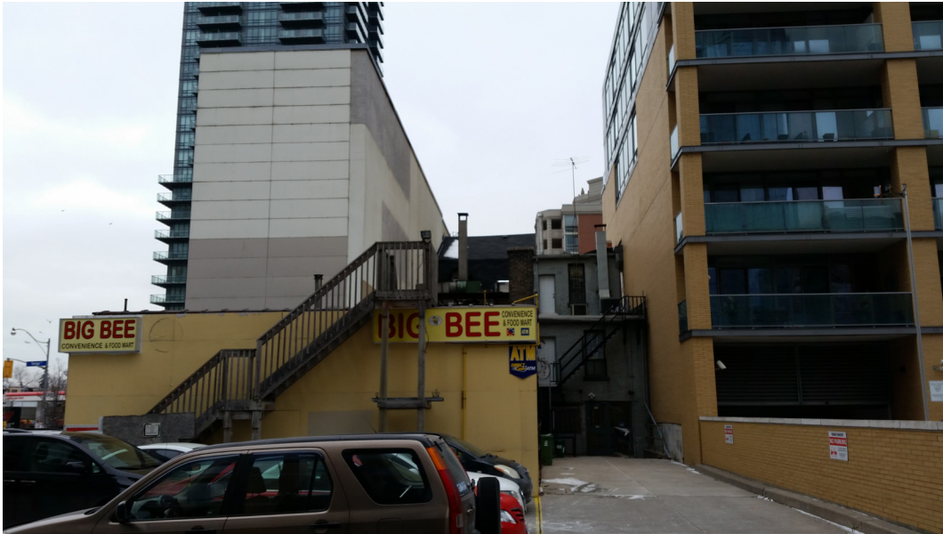
37. 874-878 Yonge Street rear elevations (Source: ERA Architects)
