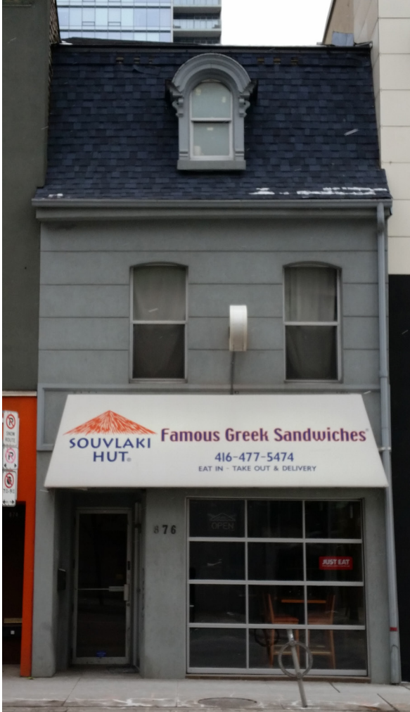
32. 876 Yonge Street (Source: ERA Architects)
