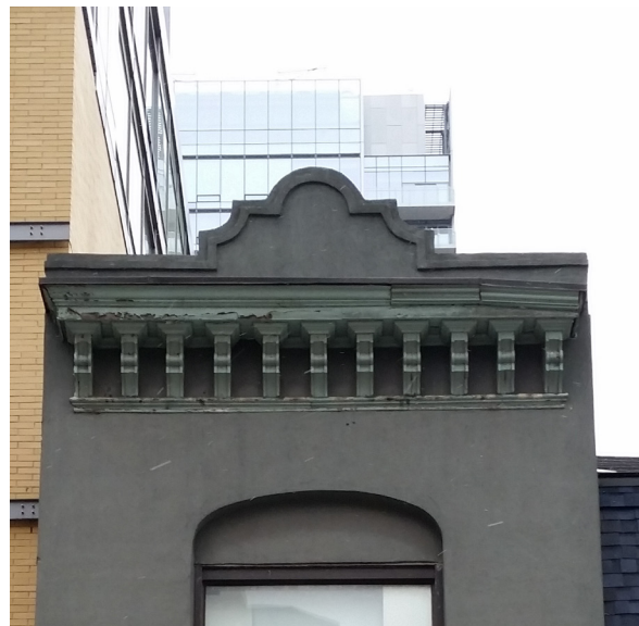
31. 874 Yonge Street (Source: ERA Architects)
