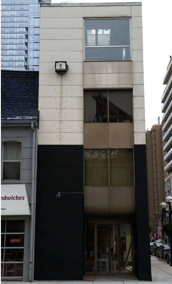
34. 878 Yonge Street (Source: ERA Architects)
