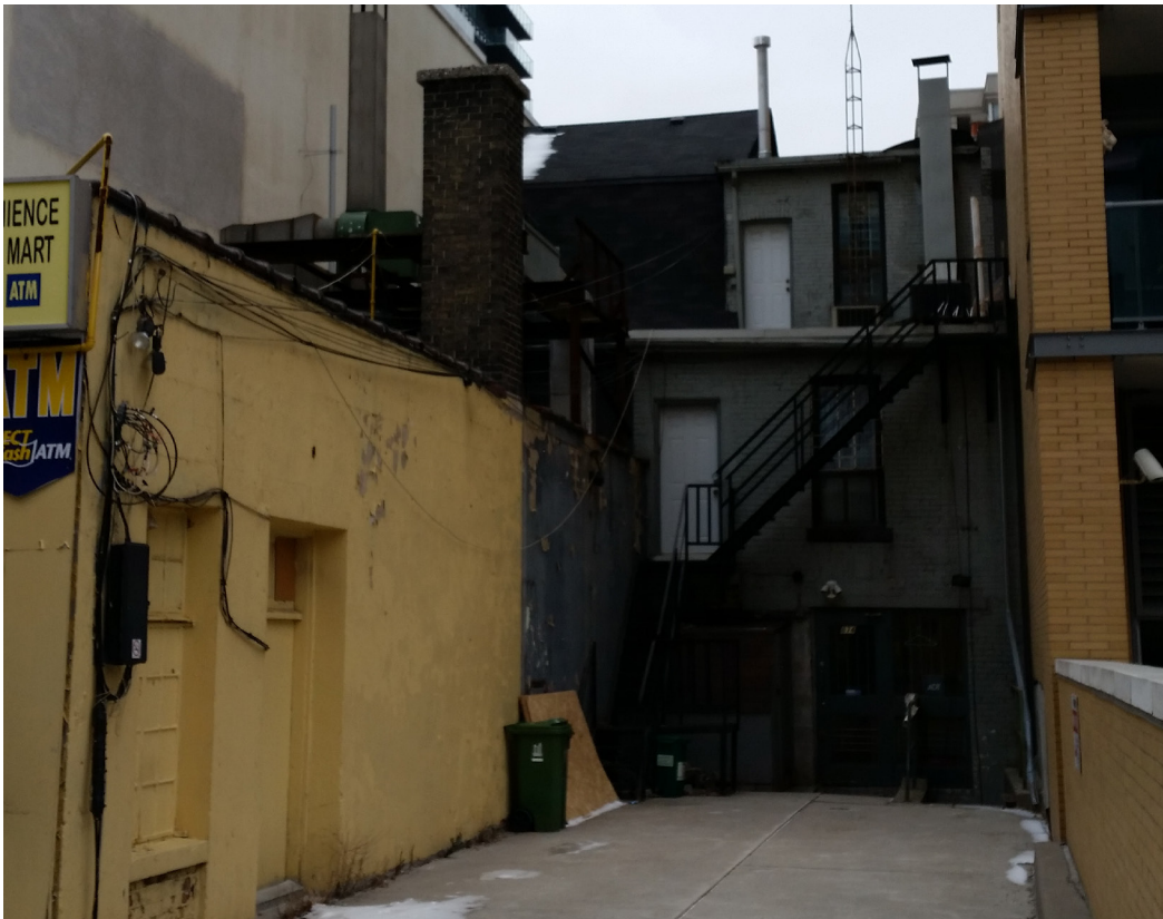
38. 874-878 Yonge Street rear elevations (Source: ERA Architects)
