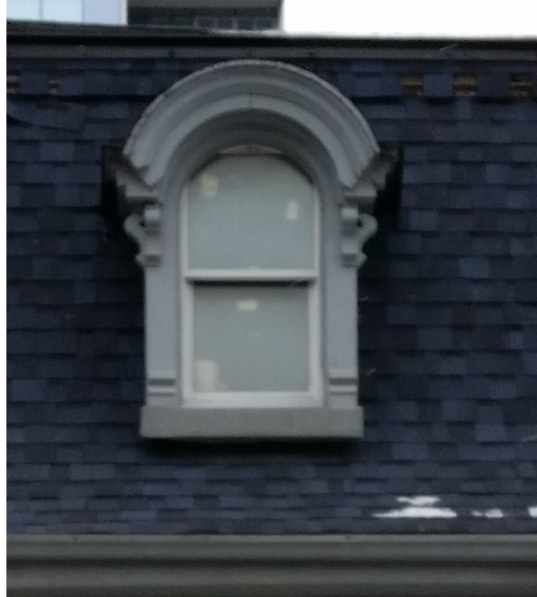
33. 876 Yonge Street (Source: ERA Architects)
