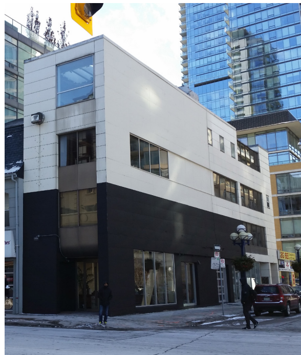
19. 878 Yonge Street (Source: ERA Architects)
