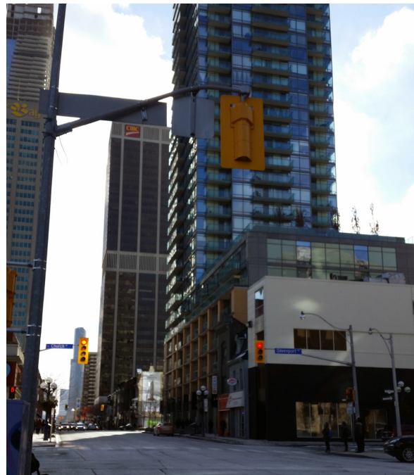
21. Context view of Subject Site from the north on Yonge Street (Source: ERA Architects)
