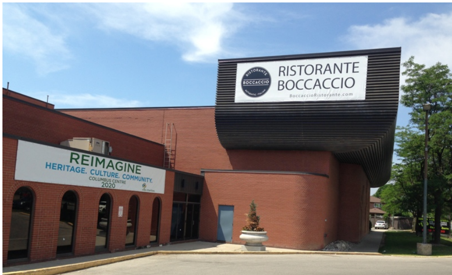
23. Looking west at the giant cornice-type element of the additional athletic facilities (HPS, 2018)
