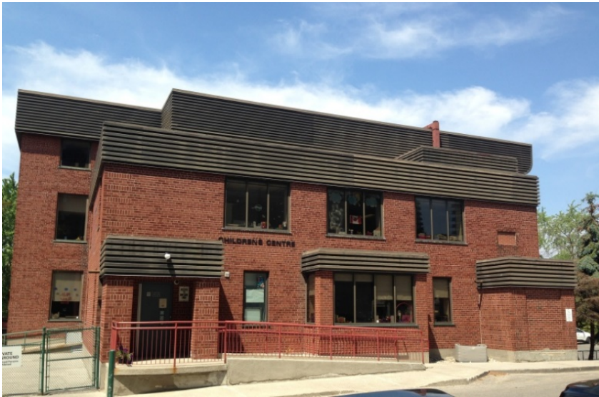
13. East Elevation, former St. Mary's Training School showing the entrance wing (HPS, 2018)
