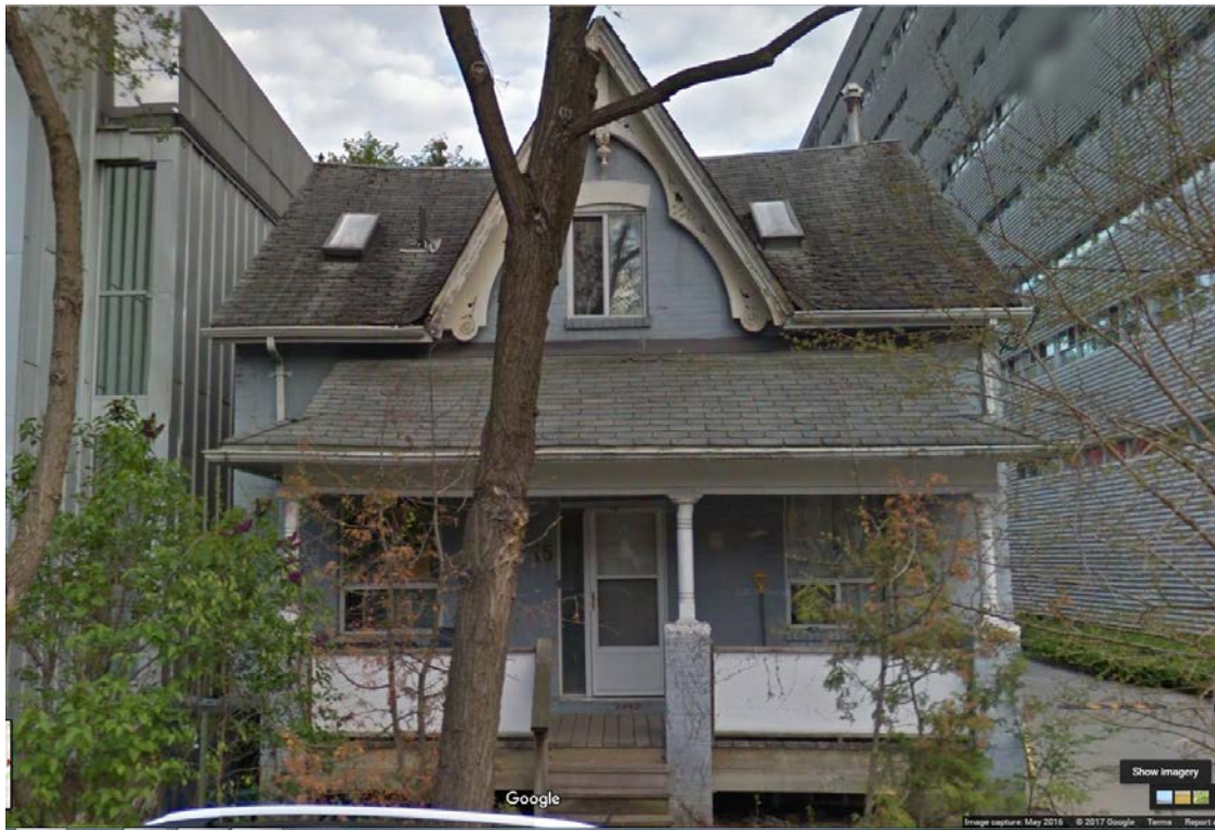
12. 15 Glen Morris Street, Photograph taken in May 2016 with the original barge-board and recent wood columns on the brick piers of the verandah (Google Maps, May 2016)
