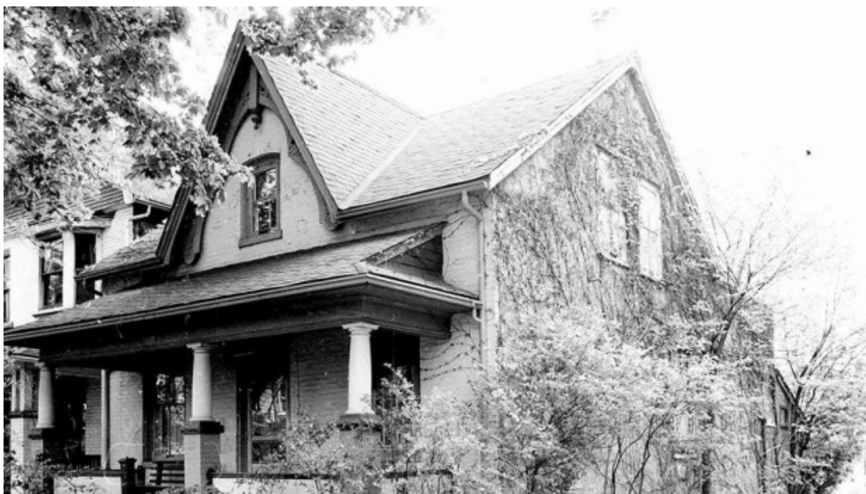
9. Samuel Bennett house, photograph from 1973 showing the verandah with its original columns, the gable bargeboard and the windows with their double hung, two-over-two sash. (City of Toronto Archives [CTA], Fonds 2043, Series 1587)
