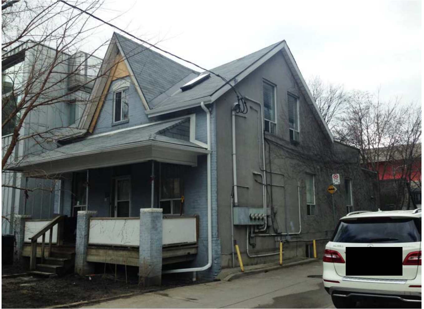
Photograph of 15 Glen Morris taken in 2017: Note the removal of the porch columns and the gable dormer bargeboard (Heritage Preservation Services [HPS])
