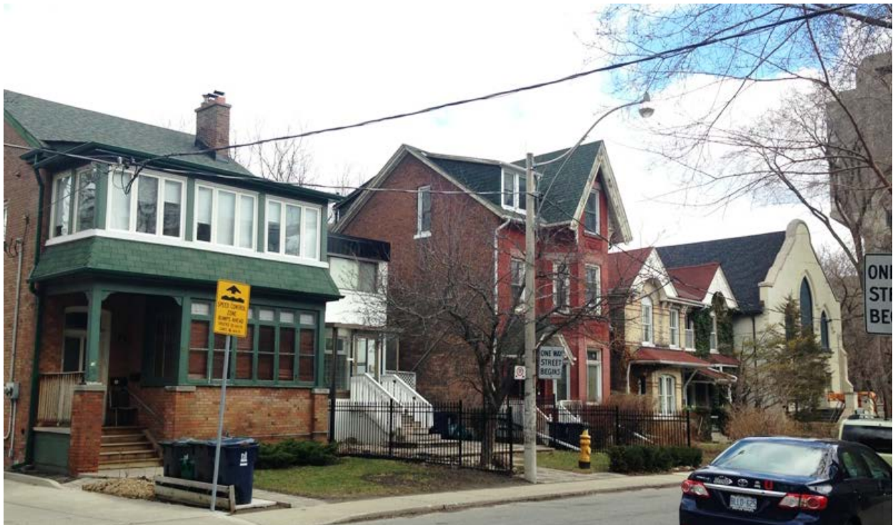
13. Late-19th century houses and the church of 1913 on the north side of Glen Morris Street. Note Roberts Library at the upper right hand of the photograph (HPS, 2017)
