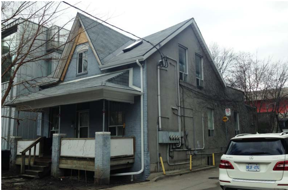
7. Samuel Bennett House, Principal (north) and side (west) elevations, showing the removal of the gable dormer bargeboard and the verandah columns (HPS, 2017)
