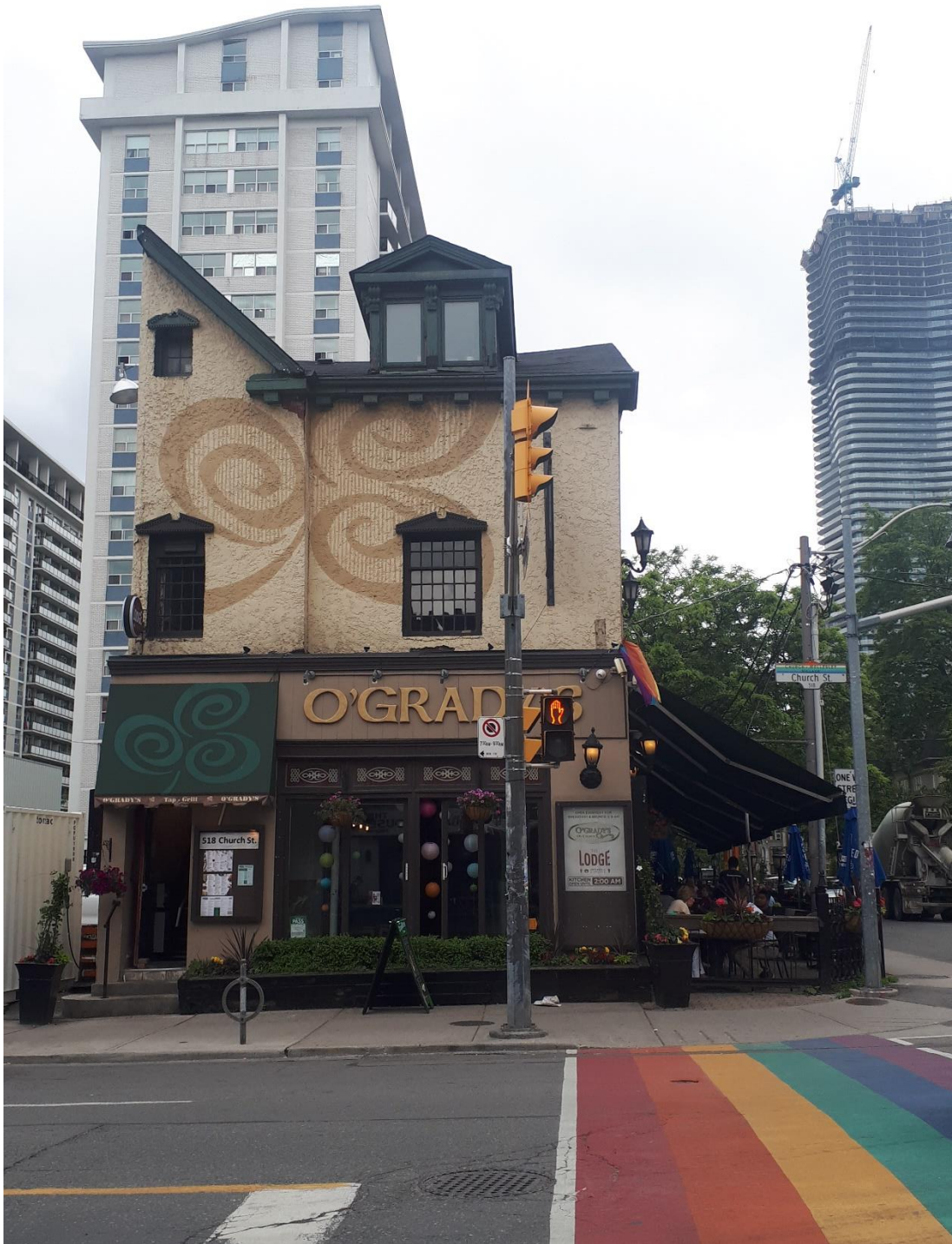
Appendix B, Figure 12 Above: 518 Church Street circa. 2019. Source: Photograph by Adam Wynne
