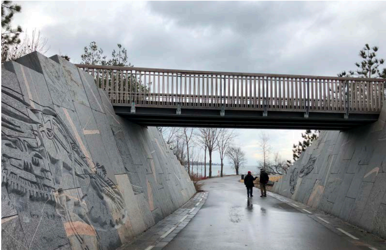
Trillium Park and William G. Davis Trail photograph showing the "Ravine" with the Moccasin Identifier carvings and the walls composed of Muskoka granite blocks. (HPS, 2019)
