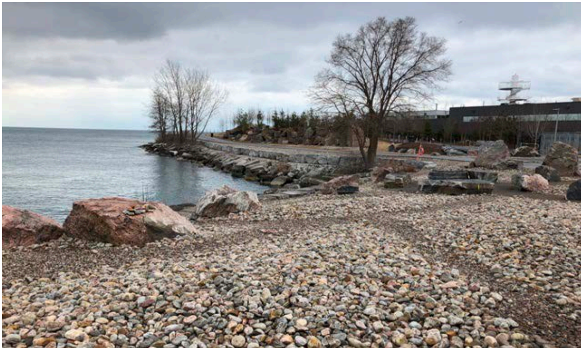
11. Looking south, the shoreline edge with its raised level and boulders to provide effective breakwater against rising water levels and flooding. The variety in stone sizes was designed to create pathways. (HPS, 2019)
