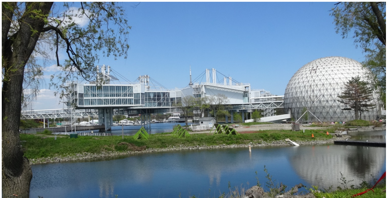
Ontario Place looking south-east and showing the Pods (centre) set over the water, linked by bridges and the Cinesphere contained in the triodetic dome. (HPS, 2015)
