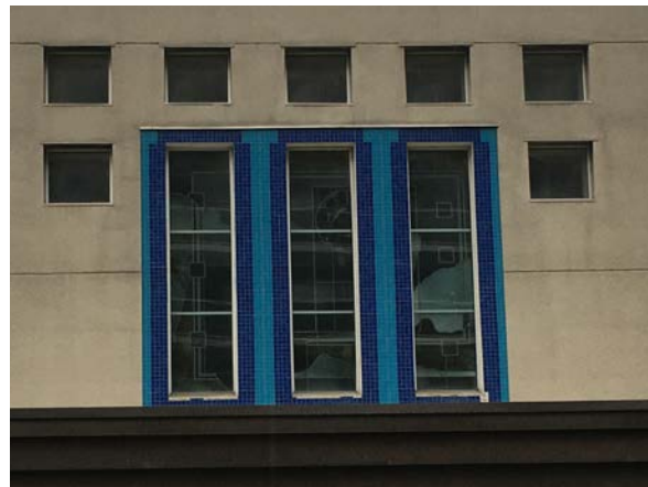
West elevation, triple windows (ERA, 2020).
