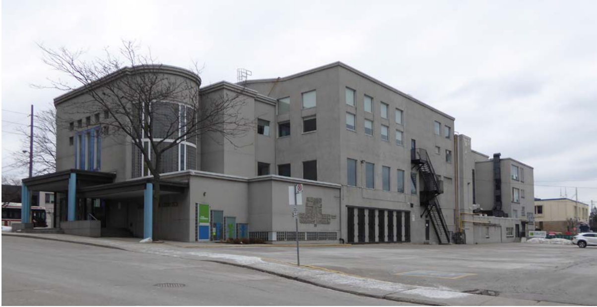
Southwest corner of site viewed from Atlas Avenue (BNKC, 2018).
