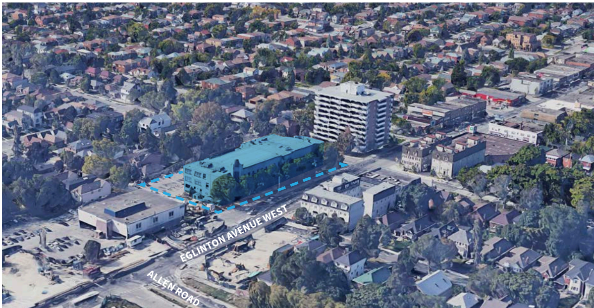
Axonometric image of Beth Sholom Synagogue with the site boundary outlined in blue (Google Earth, 2019; annotated by ERA).
