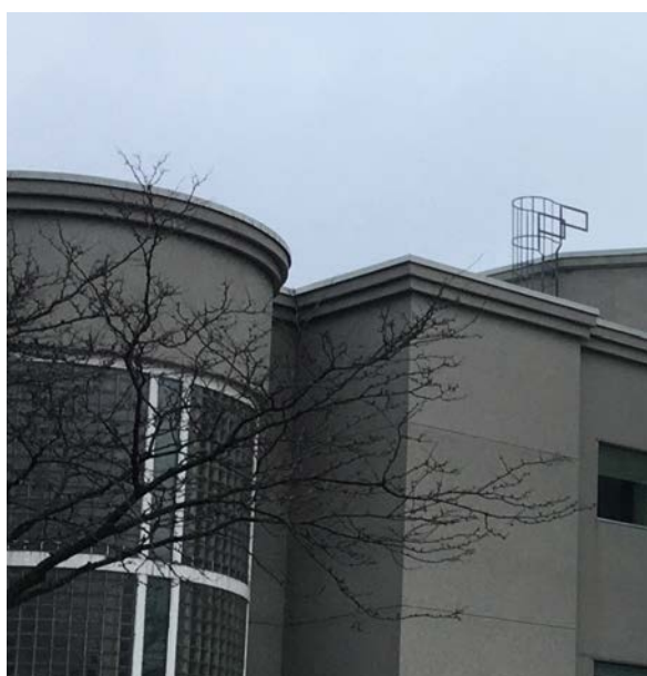
Typical condition of flashings (ERA, 2020).
