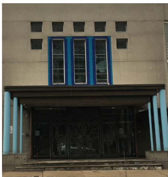
West entrance (ERA, 2020).
