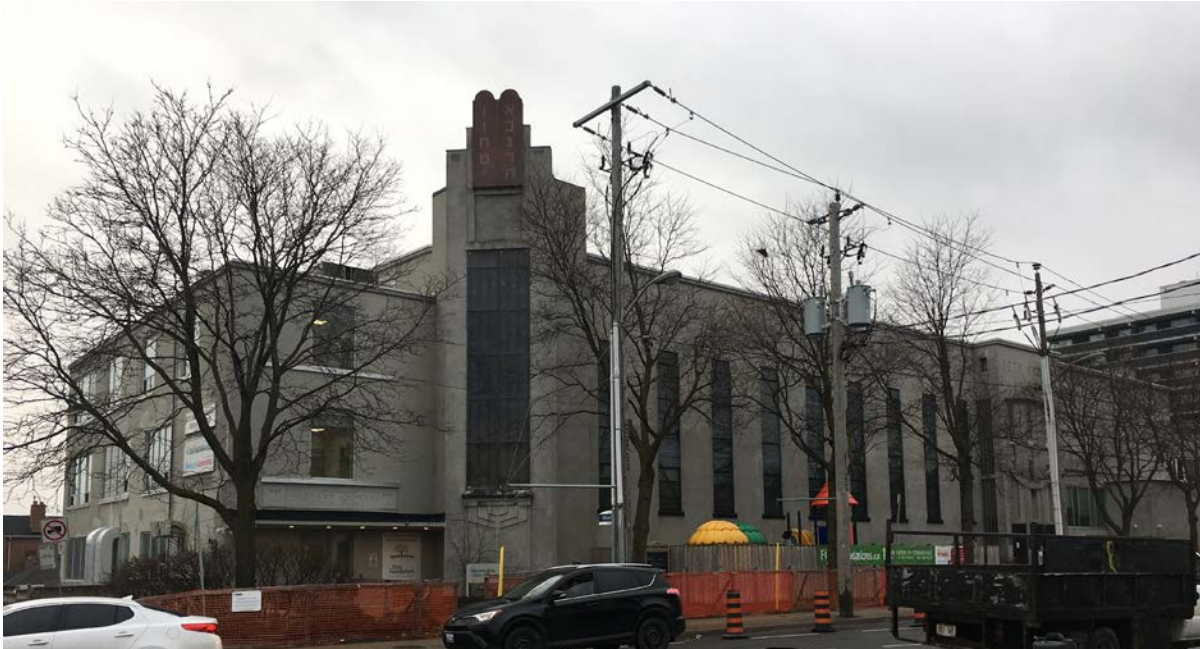
North elevation of Beth Sholom Synagogue (ERA, 2020).
