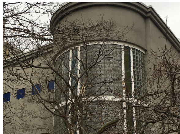
West elevation, glass block windows in curved bay (ERA, 2020).
