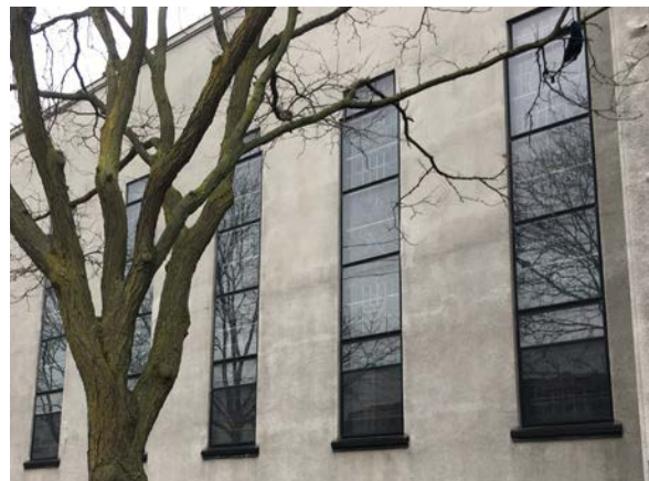
North elevation, exterior storm windows over coloured leaded glass windows (ERA, 2020).
