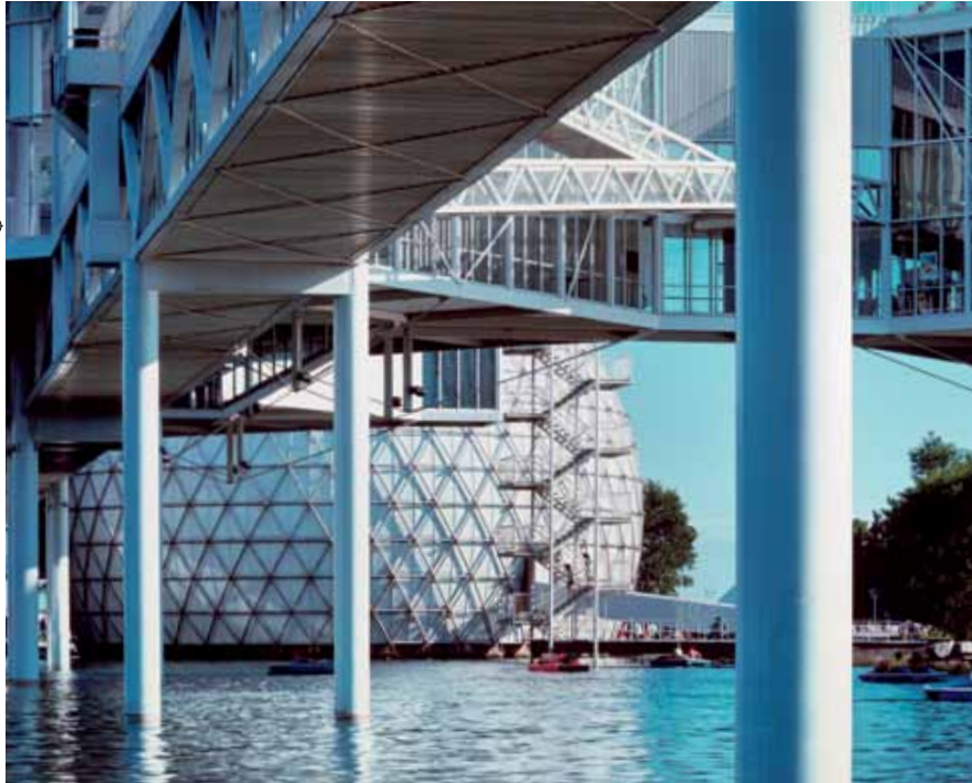
FIG. 7.8: Ontario Place, Toronto, 1968–71. Tensile construction and bracing.
