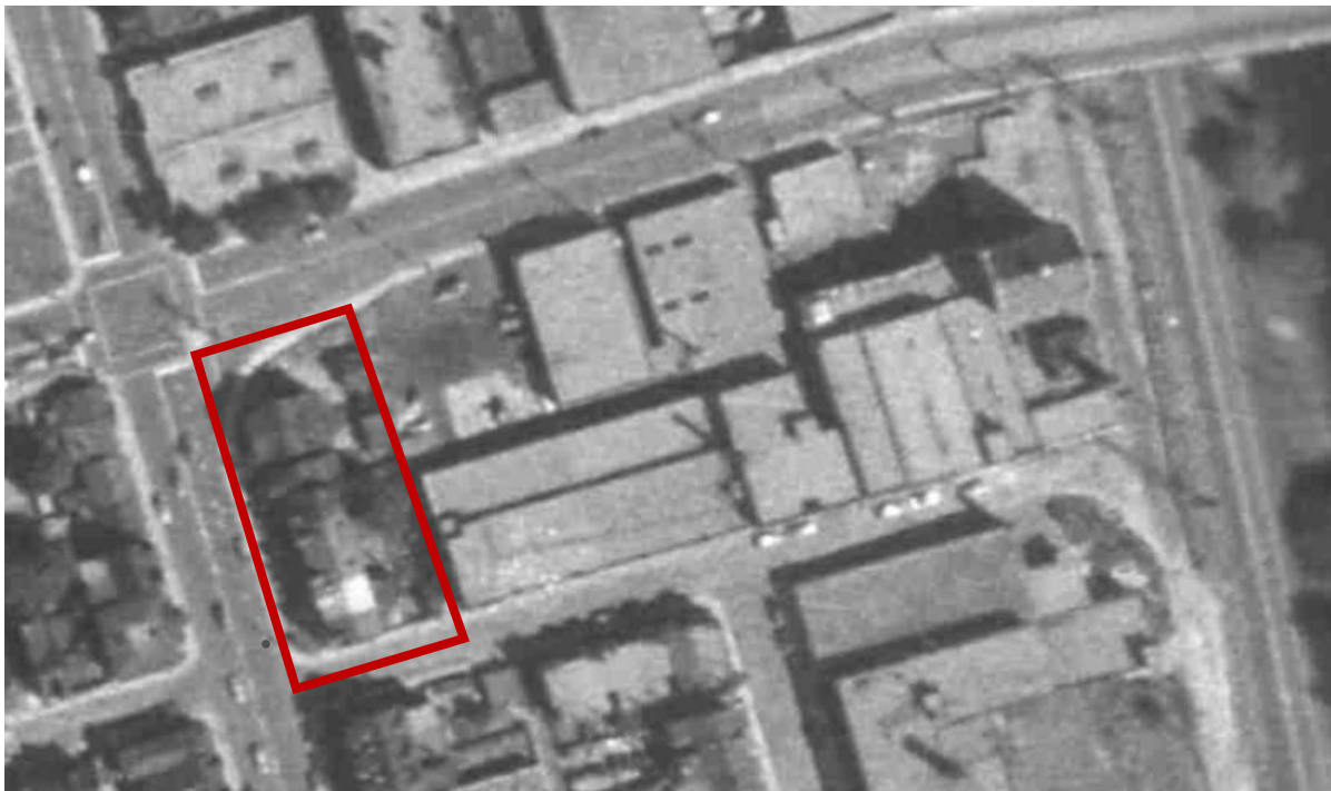
Figure 9. 1954 aerial photo showing the southeast corner of Dundas Street East and River Street after Dundas Street East was realigned. This resulted in the demolition of 127 and 129 River Street and alterations to 123 and 125 River Street (City of Toronto)
