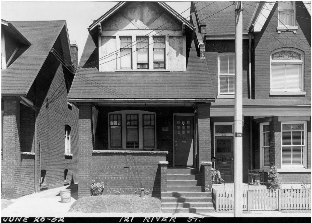
Figure 10. 1952 historic photo of 121 River St (left) and partial view of 119 River St (right) showing both properties prior to alterations (City of Toronto Archives)
