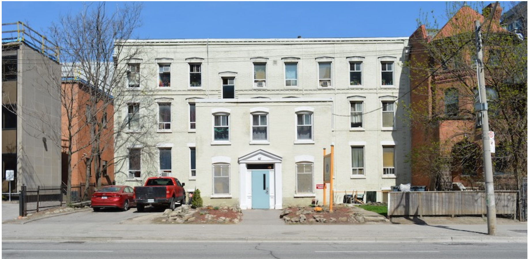
West (main) elevation of the Inglewood Arms Hotel at 295 Jarvis Street
